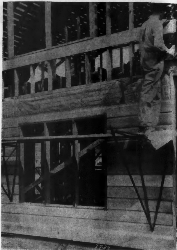
The Cooper Homes Were Constructed with Eel Grass Insulating Material. This feature is appreciated by buyers, it has been found.
