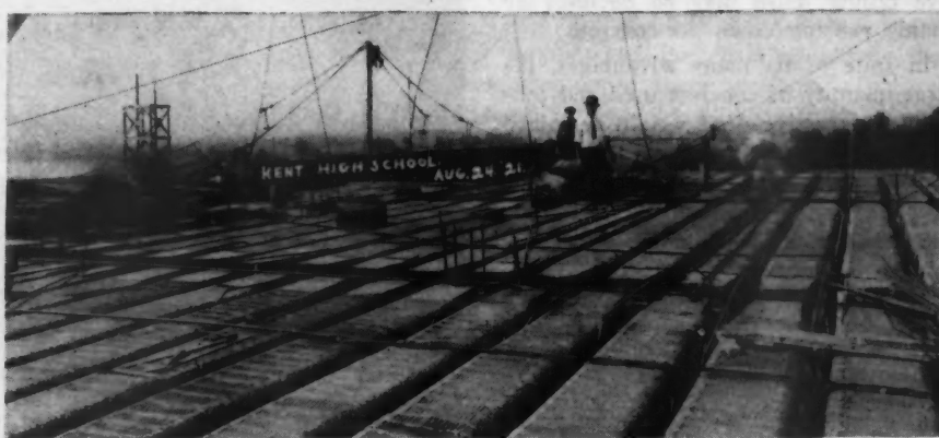
Steel Tile Used in Construction of Kent High School, Kent, Ohio.
