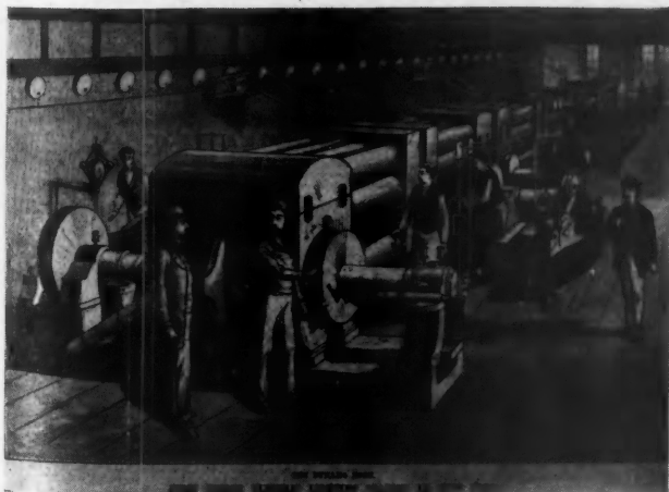
"Jumbo" Generators in the First Central Station, 255 Pearl Street, New York City, Opened Sept. 4, 1882.
