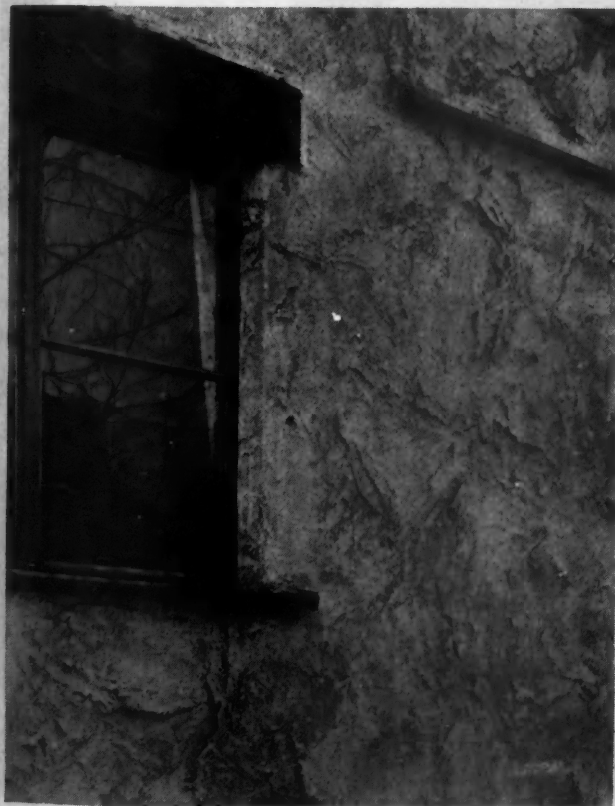
Close Up View of Characterful Stucco Finish; Also Note That Zinc, in the Form of Small Squares, Was Nailed to the End of Every Window Sill to Prevent Concentration of Water and "Tear Stains" or Streaks on the Stucco Below.
