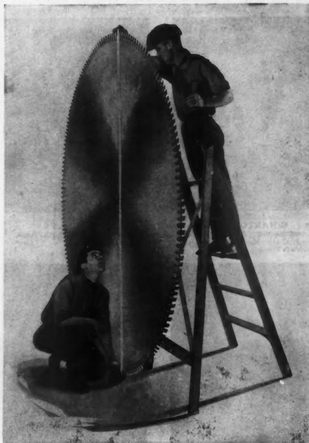
Type of Giant Size Circular Saw Now Employed in American Saw Mills. This one of the inserted tooth variety measures 108 inches in diameter, the largest yet made.
