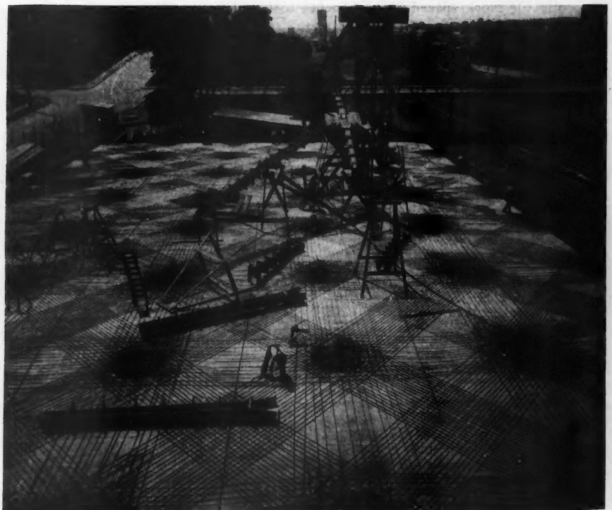
Flat Slab Construction—Reinforcing Steel in Place Before Concrete is Poured.
