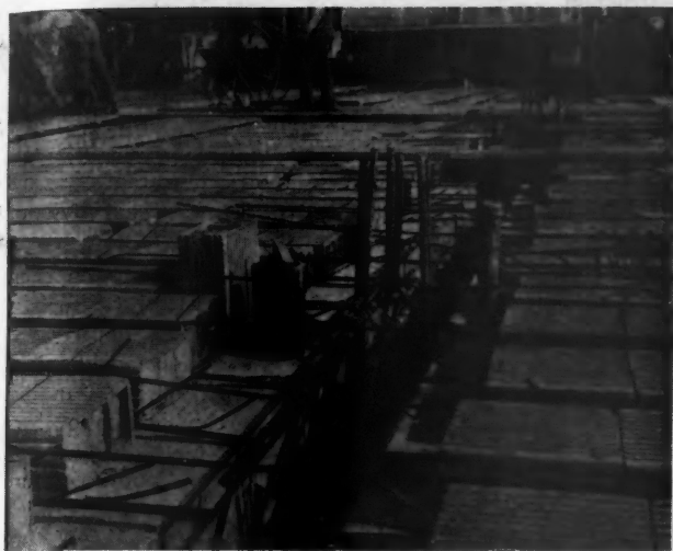
Concrete Joist and Clay Tile Construction.
