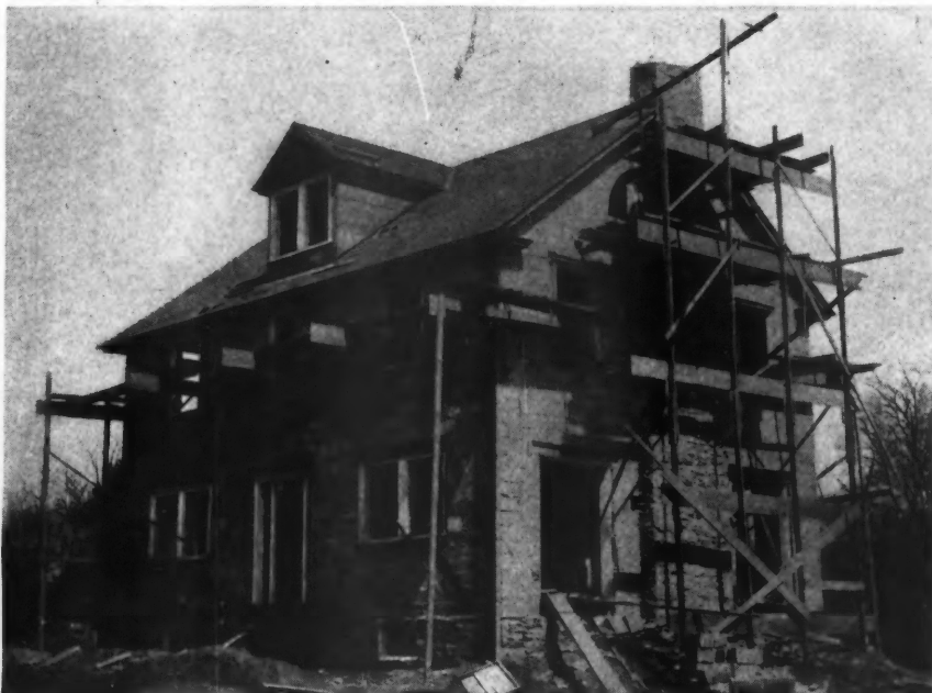
Concrete Blocks Ready for Stucco Finish.
