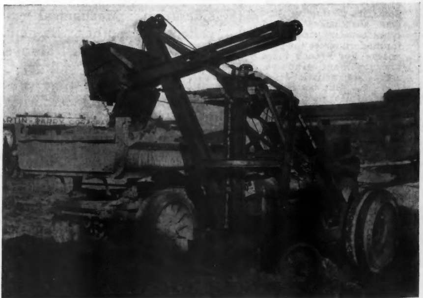
For the Builder Who Handles a Large Amount of Gravel, Crushed Stone or Other Material of a Like Nature, This Power Shovel Will Prove Useful. It also can be used for light excavating work.
