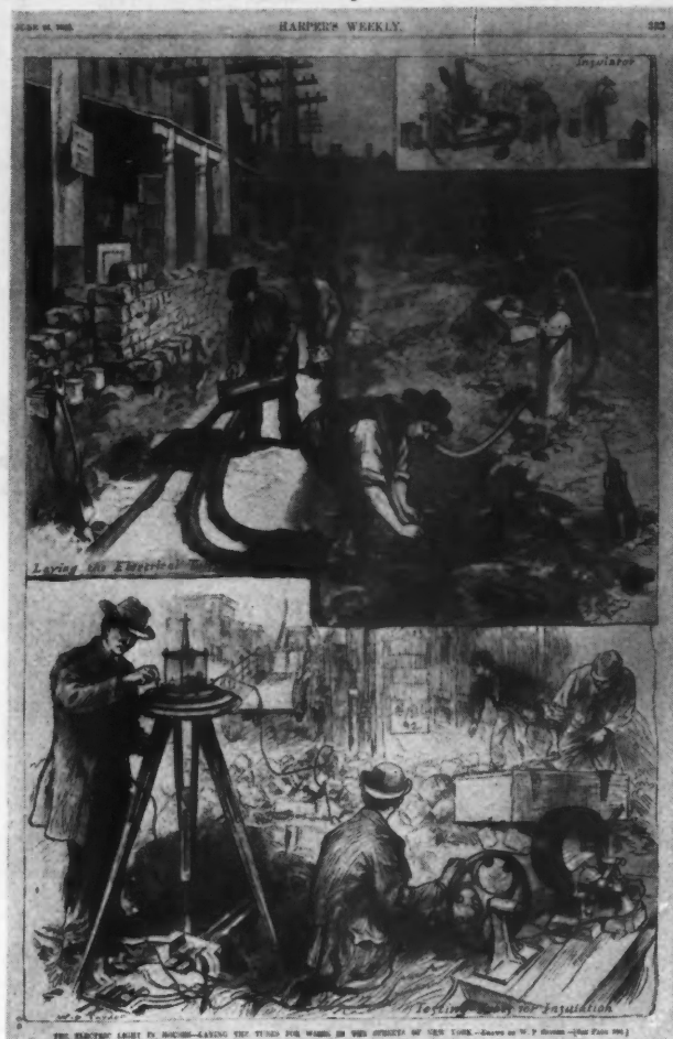
Laying the Underground Conductors for the First Central Station, New York City, 1881-1882.
