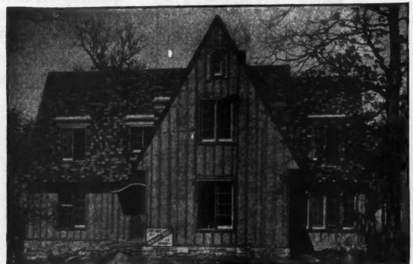
House near Chicago, showing us "underclothing" of Cabot's Quilt, with jurring strips over the Quilt, on which the outside finish is laid. Roof also insulated. Leon E. Stanhope, Architect, Chicago.
