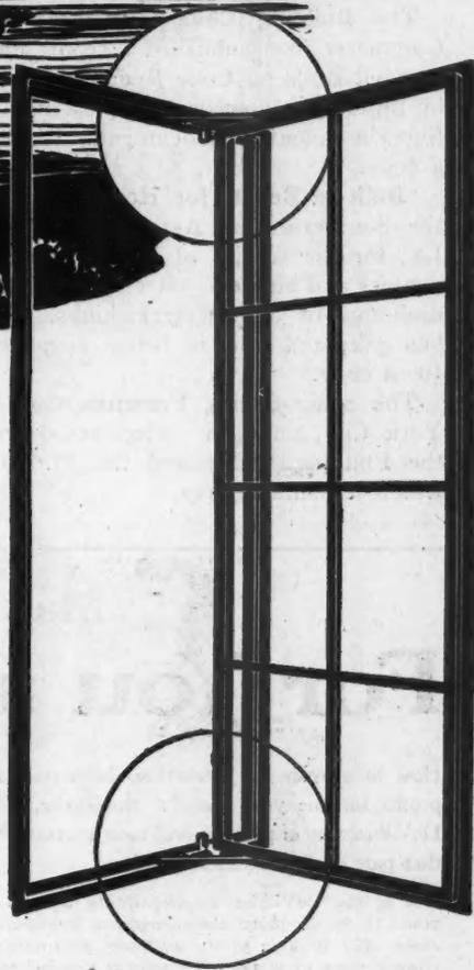
*Notice how this friction control at both top and bottom of a Thorn casement holds the leaf open firmly at any position*
