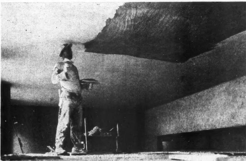
**Applying the Brown Coat of Acoustical Plaster Over Half-Green and Scratched Base Coat of Gypsum Plaster. The application of this plaster is practically the same as that of ordinary plasters.**
