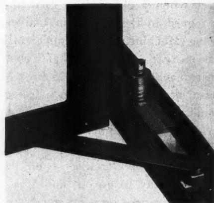
**The Vital Portion of This New Steel Casement Sash Is the Original, Sliding Hinge Construction Shown Here.**
