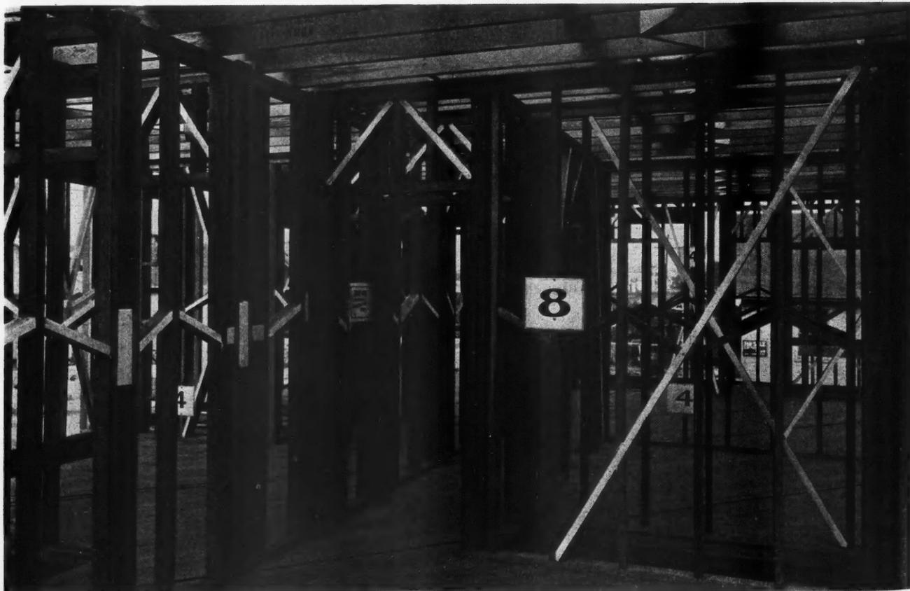
General Interior View. The thickly clustered studs usually indicate where a partition or wall joins another, forming a vertical slot into which the walls, or partitions, fit and are blocked and spiked into position. Tying of walls to partitions and partitions to one another, is one of the urgent requirements for safety under powerful hammering and twisting storm stress.
