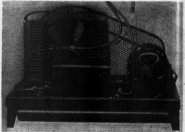
Here Is the Compressor Unit for the Drinking Fountain Shown at the Left. It can be placed in the basement or anywhere within 50 feet of the cooler.
