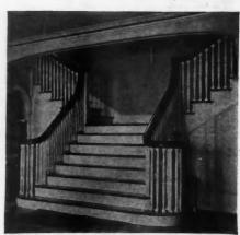
Millwork plants are turning to Douglas Fir and duplicating the results they used to get with the old-time. White Pine. Here is some Douglas Fir millwork.
