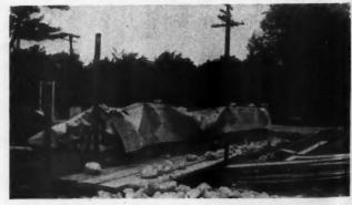
This Building Paper Is so Tough That After Being Used to Protect the Foundation It Was Still in Condition for Use in Sheathing.
