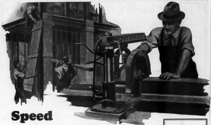
YOU can set early completion dates without fear, when your equipment includes a DeWalt. Speeds the job all along the line, from the shoring of the excavation, and the concrete forms, to the room trim. Use it right on the spot. Runs from any lamp socket. Two men can easily carry it anywhere. Tools changed in 30 seconds. Direct drive—no wobbly belts.
