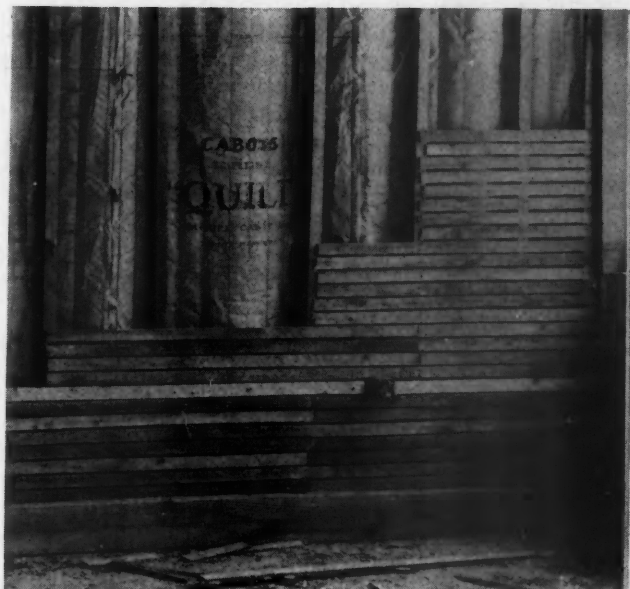
The Insulation Here Shown Between the Studs of a Wall Under Construction Is Made of Marine Grasses Quilted Between Sheets of Waterproof Paper. This insulation is impervious to moisture and has excellent insulating qualities.
