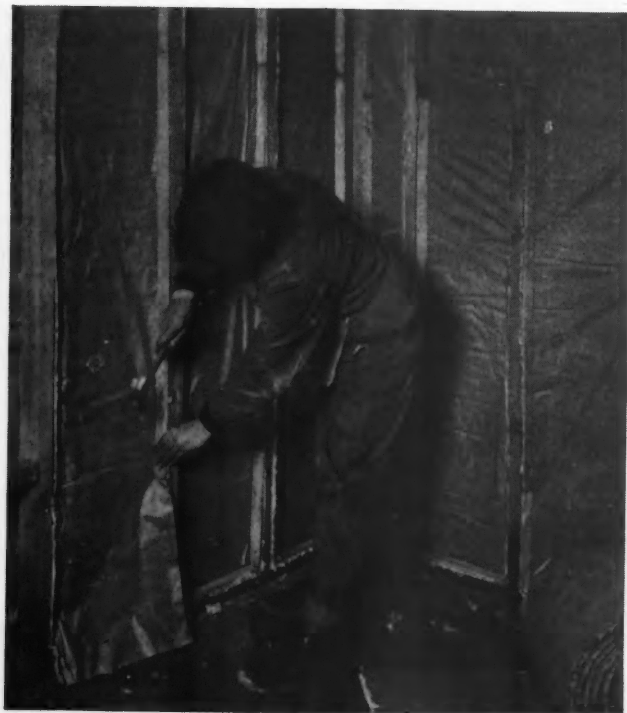
The Insulation Here Shown Is a Wood Fibre Quilted Between Sheets of Special Paper and Is Being Nailed to the Studs Under Lath Strips. A roll of the material, revealing its fleecy nature, is seen at the right.
