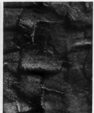
ENGLISH A soft, heavy texture applied with wood float and brushed
