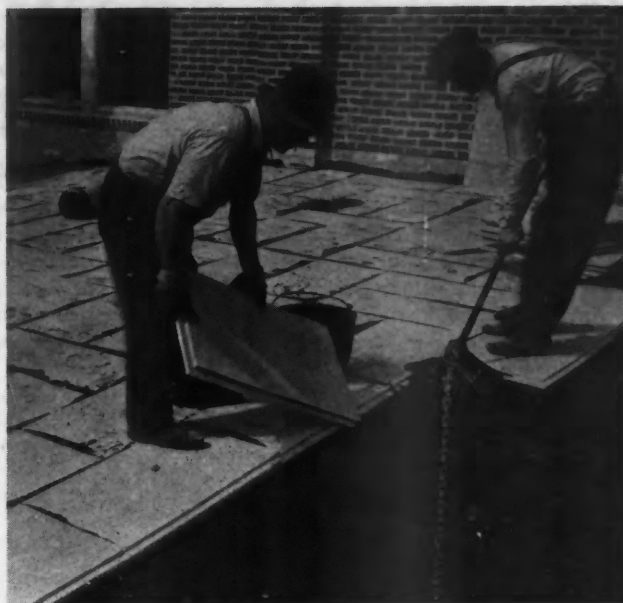
Here We See the Insulation of a Concrete Roof Deck with Sheets of the Pressed Wood Fibre Type. This insulation is mopped over with hot asphalt as a top finish. It prevents excessive heat loss and condensation or drip underneath.
