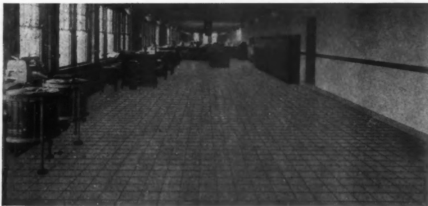
Employers Have Learned the Value of Good Finish, Bright and Clean Surroundings in Factories and Workshops as Well as Offices. Note the well finished, sanitary appearance of this plastic magnesia flooring laid in tile pattern.
