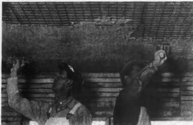
As a Plaster or Stucco Base This Material Gives Excellent Results Assuring an Effective Reinforcement.
