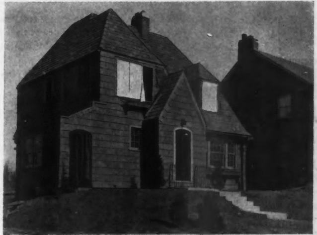
After the Fire—Note that the Exterior Is Undamaged Although the Inside Was Burned Out Clean. Gypsum filling between the studs stopped the fire.
