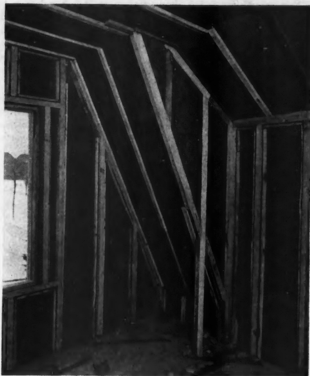
The Insulation Used Between the Studs in This Picture Is Made from Flax Fibres Felted and Pressed Into Semi-Rigid Sheets. It has good heat resisting qualities and is non-inflammable.
