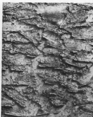
ENGLISH COTTAGE A fine, leaf-like finish produced by feathering with trowel
