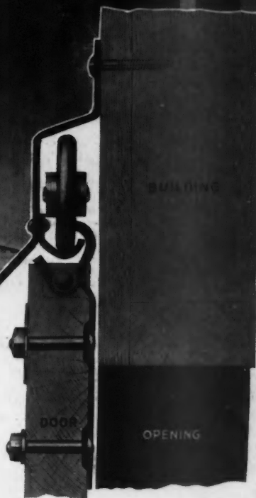
The FIRST installation of "Glide" Hangers and Track was made in 1911, on the John Phillips Farm, west of Dixon, Illinois. After 16 years of service the Track is intact and the Hangers are still carrying the door with the same ease and smoothness as when new.
