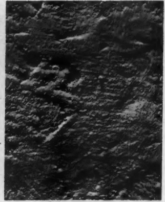
ROUGH CALIFORNIAN A rough cast finish reduced by rubbing with a carpet-covered float
