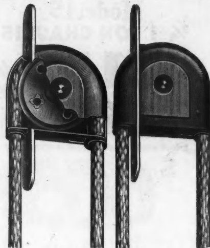
Improved Sash Pulley Cut Away to Show Construction.
