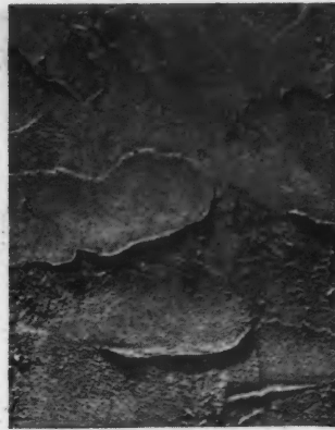
ENGLISH The irregularities are produced by side strokes of the trowel
