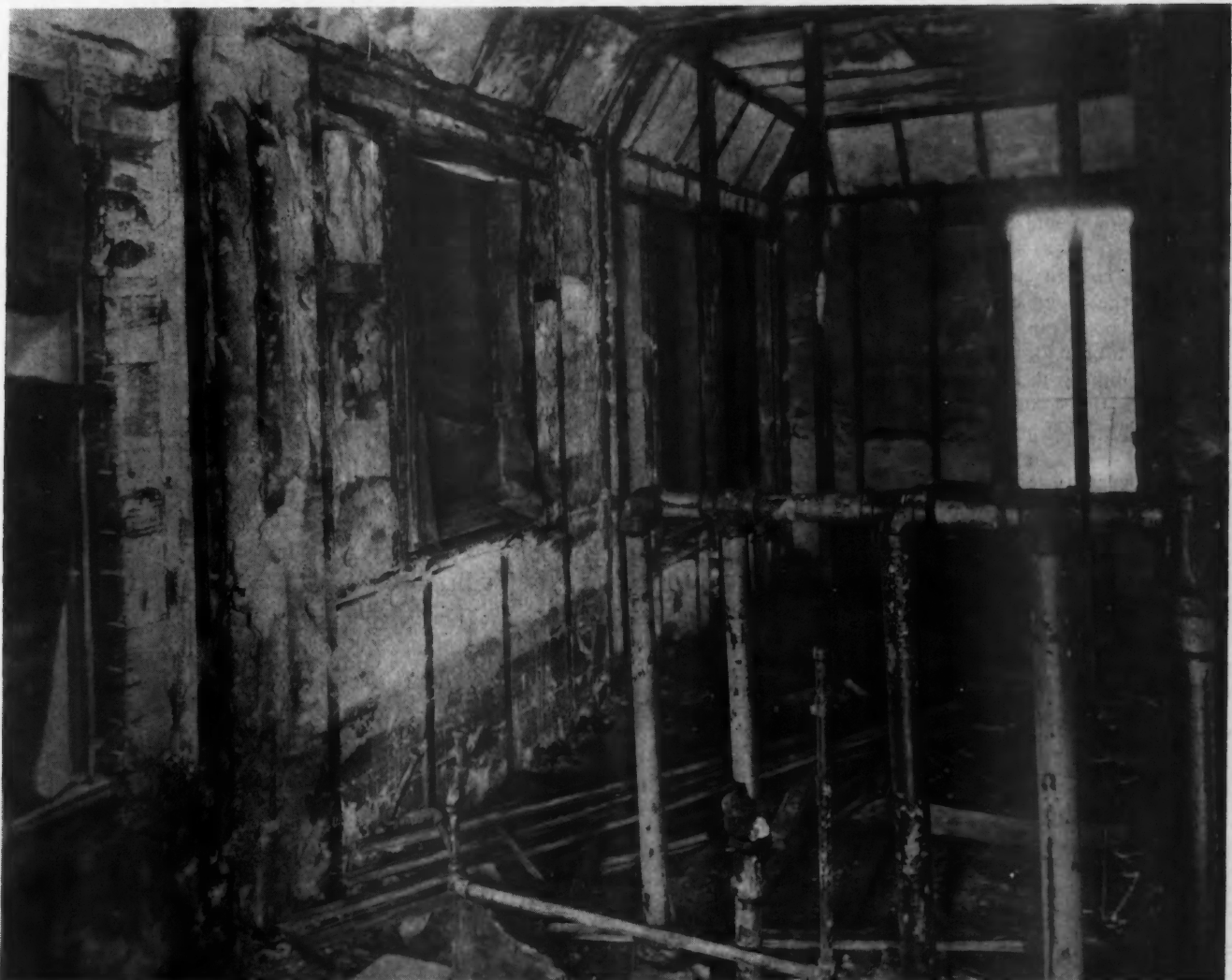
After the Fire—Inside Partitions and Outside Wall Lining Completely Burned; Edges of Studs Charred; Gypsum Insulation, Which Stopped the Fire, Still in Place.
