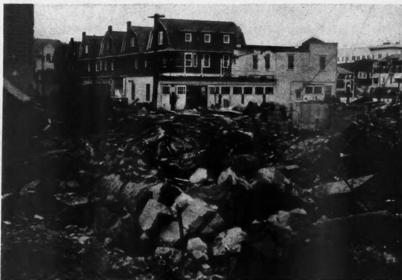
The Office of a Garage, Covered on the Sides with Asbestos Shingles, Acted as a Fire Stop When the Main Garage Burned, in the Recent Fire at Ocean City, N. J., and Also Prevented the Loss of the Six Double Frame Houses Beyond.
