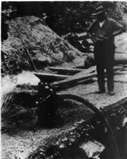
This Centrifugal Pump Weighs But 95 Pounds, But Has a Capacity of 7,500 Gallons an Hour.
