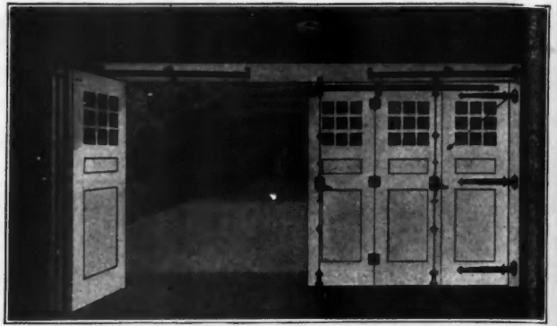
Operating Arms for Multiple Doors Are Made in Two Sizes and Are Adjustable to Series of Three or Four Doors Folding One Way.
