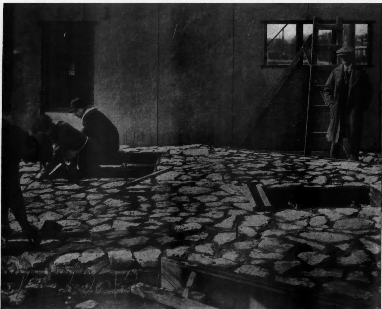
In the Foreground, Unskilled Workmen Are Embedding Stone Slabs in the Soft Mortar to Make the Outside Decorative Face of One Side of the House. In the background we see the inner face of the adjacent side wall, already raised.
