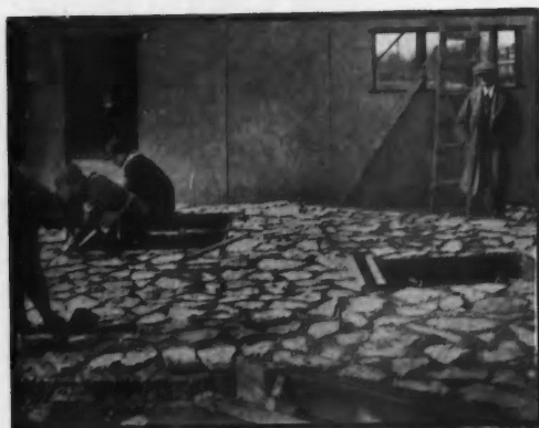
The photo above shows how Tri-Ply walls are built lying on a flat surface.
