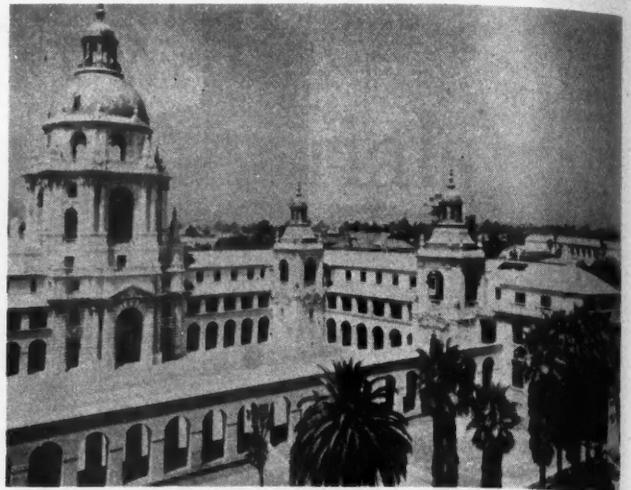
City Hall, in Pasadena, California, Roofed with Lead Coated Copper Which Will Last Indefinitely.
