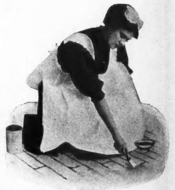
Putty That Is Mixed with Water Is Satisfactory Permanent Filling for Cracks and Crevices.
