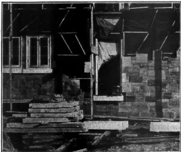
Showing how Indiana Limestone is laid up as an irregular or random veneer or facing. No carefully prepared drawings are needed.
