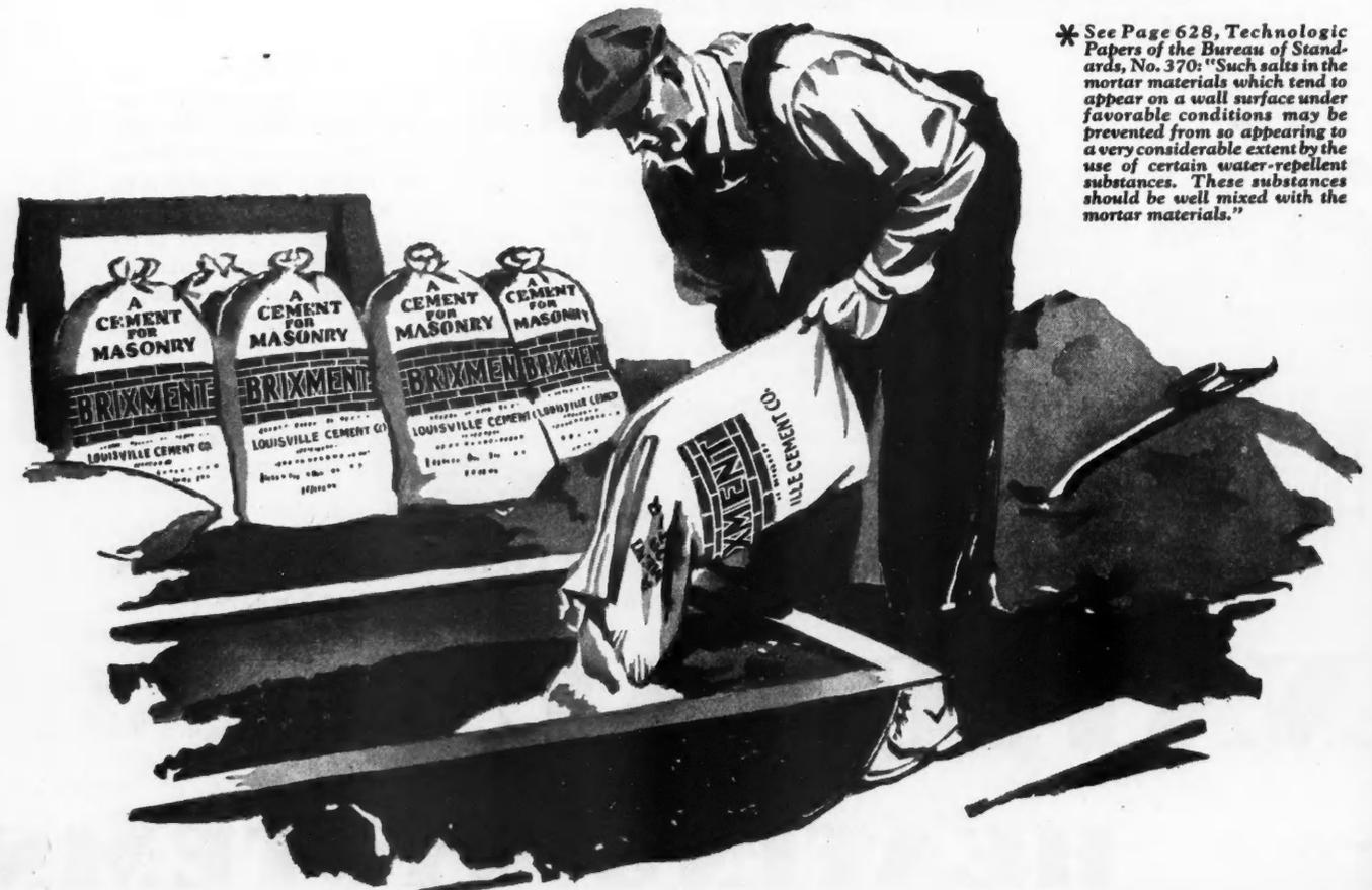
\* See Page 628, Technologic Papers of the Bureau of Standards, No. 370: "Such salts in the mortar materials which tend to appear on a wall surface under favorable conditions may be prevented from so appearing to a very considerable extent by the use of certain water-repellent substances. These substances should be well mixed with the mortar materials."
