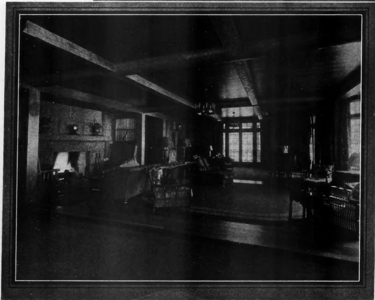
Living room, with floor, walls and ceiling of cypress and beams of birch. The transverse logs were hollowed to fit around the steel beams which support the upper floor.
