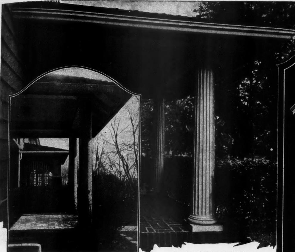
Old type columns which deteriorated rapidly and had to be replaced. Note how the joints opened.
