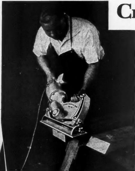
The Crowe Safety Beveling Saw always maintains its record-breaking speed—the gears will not heat, and the saw cuts on the bevel with the same rapidity with which it crosscuts.
