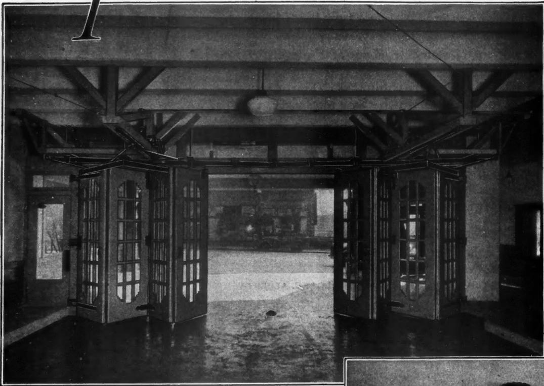
*Capitol Garage, Kansas City's largest, NEVER keeps a patron waiting. Only R-W equipment assures such service. These doors close weather tight. They open INSIDE so ice and snow NEVER hinder operation. A simple adjustment allows for swelling or shrinking of doors. No center posts. The same R-W advantages for doorways up to 30 feet wide.*
