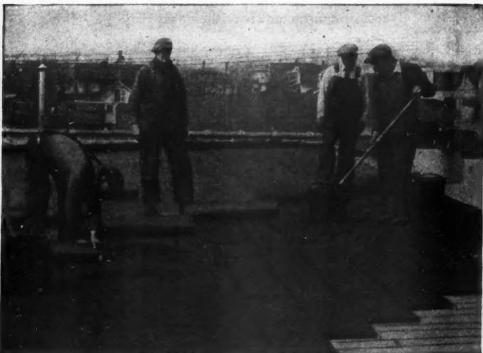
Rigideck, the light weight, fireproof roof deck. Laid like boards. Made of rust-resisting Armco Ingot Iron.
