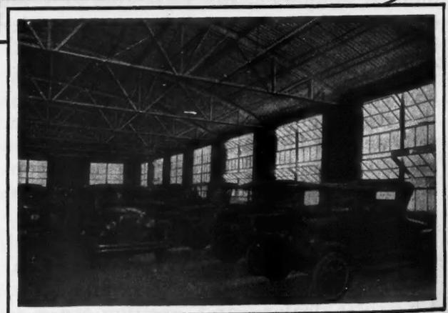
(In Oval) E. S. Koon Warehouse, Asheville, N. C. Massillon Roof Trusses in position ready to receive purlins. S. Sternberg & Co., Engineers.
