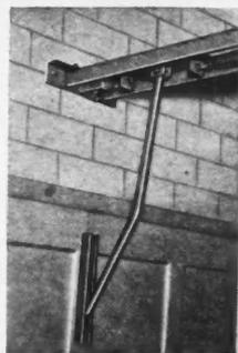
Carrier Track and Lifting Arm—Commercial Door Operator
