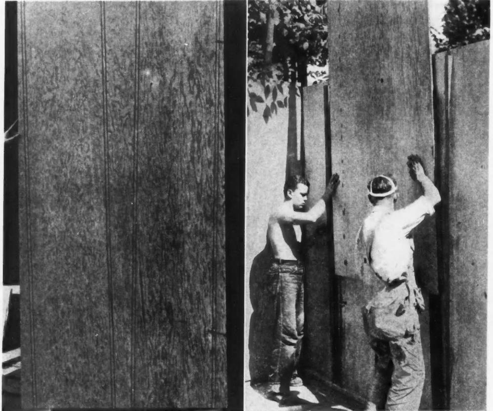
the form of an all-day down-pour. All of the panels, including the sub-flooring, however, came through this storm without the slightest trace of buckling, blistering, shrinkage, or other weakness, a fact that augured well for the adequacy of this new type of construction.
