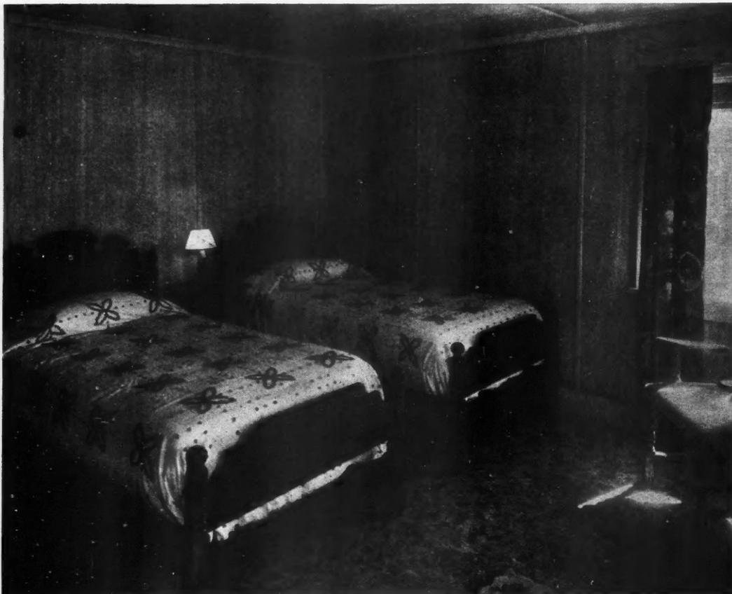
**NATURAL** finished Douglas fir plywood with grain softened by sealer priming. Wall panels have simple battens over joints—an extremely economical application.
