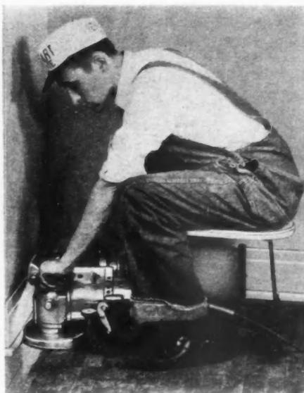
**DISC SANDER** supplements the work of larger floor machines at edges and in corners.
