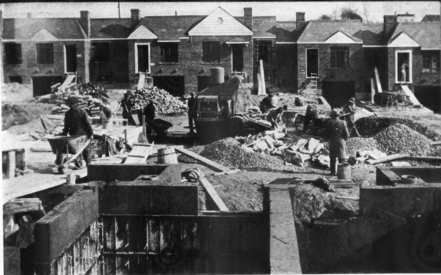
A MODERN CONCRETE MIXER, steel forms, rubber-tired wheelbarrows contribute to lower cost, better quality concrete at Green Park Homes, a successful row house project near Forest Hills, L. I. BELOW Lightweight Safety Saw with plenty of power, equipped with duplex handle for convenience in any position; cuts 2-inch dressed lumber. Scaffold brackets are time and material savers.
