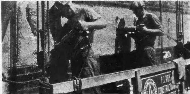
F. J. ROMER COMPANY, St. Paul contractors, saved 75 percent in direct labor cost in cutting out concrete with electric hammers.
