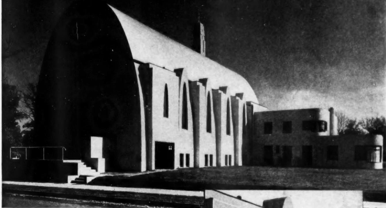
● Stucco helps to beautify St. Austin's Church and Parish House in Minneapolis. Atlas White was used in the stucco finish coat. Two under coats were portland cement stucco over expanded metal lath attached to frame construction. Architects—Bard and Vanderbilt, Minneapolis. Contractor—Herman Jeub.
