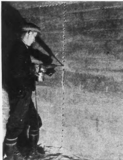
ELECTRIC HAMMER with concrete drill bit simplifies job of cutting openings in wall.
