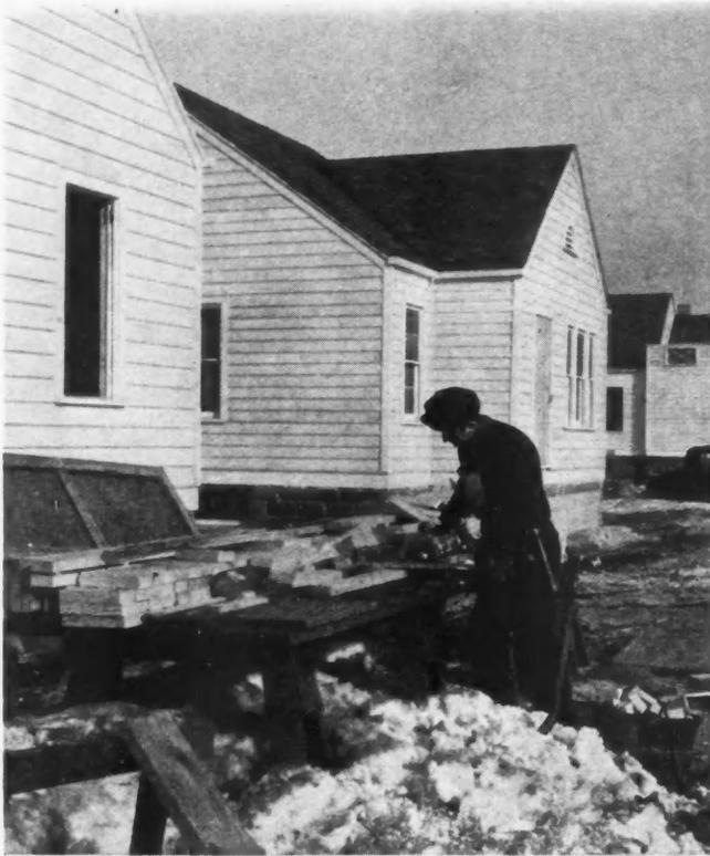
CUTTING of window framing with power hand saw is fast and accurate on Hammond, Ind., project even in cold winter weather.
