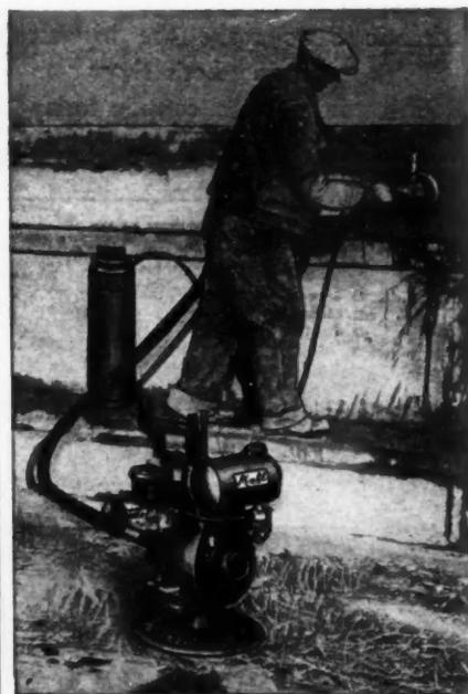
FOR surfacing, finishing, drilling and brushing concrete surfaces, a new light-weight gas engine unit offers speed and wide utility.
