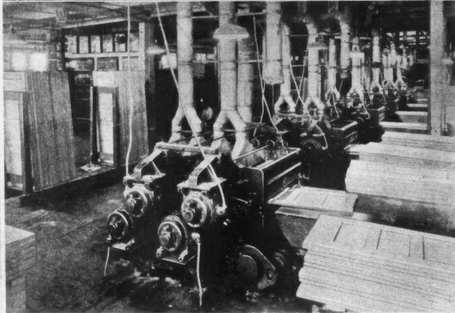
of highly accurate boring and 3-in-1 doweling machines, together with the use of high grade improved glues as bonding agents, has brought added strength and rigidity to stock doors far beyond actual requirements in use.
