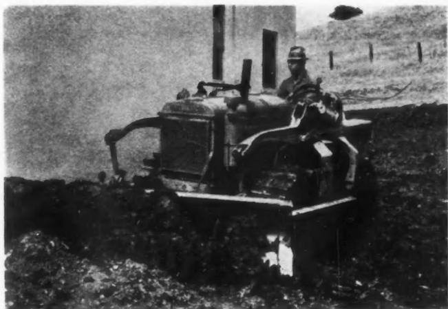
**BULLGRADER** mounted on a tractor speeds the work of Contractor Ted Oliveira, Lafayette, Calif., on the excavation for the basement of Orinda Public School. Backfilling and grading are also simplified.
