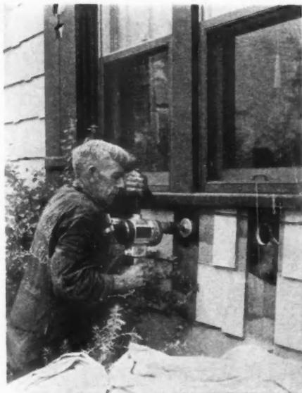
**ROTARY HACK SAW** attached to power drill is used on walls to cut holes up to 3 1/2".
