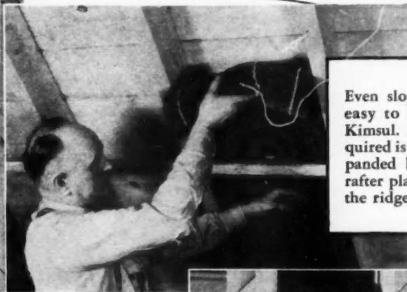
Even sloping roofs are easy to insulate with Kimsul. All that is required is to fasten an expanded blanket to the rafter plate, pull taut to the ridgepole, and nail.
