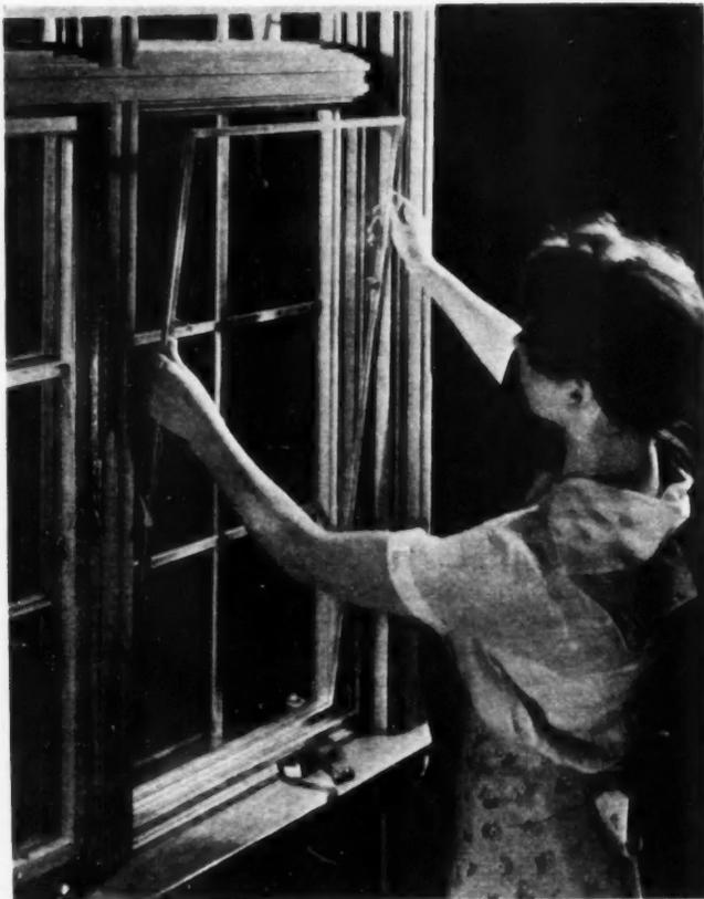
**STORM SASH** comfort (above) from accurately fitted unit windows. Today this health protection is not an afterthought but is provided in the window assembly as it comes from the manufacturer. **BELOW** is shown the modern inside storm window for wood casements. Manufacturers advise leaving them on the year round. They're installed in a jiffy. Complete with spring leaf weatherstrip, they swing with the sash.
