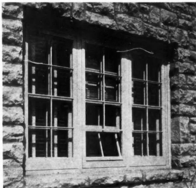
CURTIS "Silentite" double hung windows with prefit "Protectorvent" storm sash in place. Note narrow mullions which give streamlined effect. "Silentite" fits any wall construction—is made in all commonly used sizes. Sash available in several styles.
