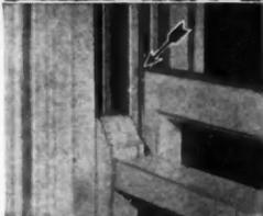
Side jambs completely metal clad from inside stop to blind stop. Upper sash is slide-sealed to metal covered parting stop with special interlocking metal strips. A complete weather and dust seal.
