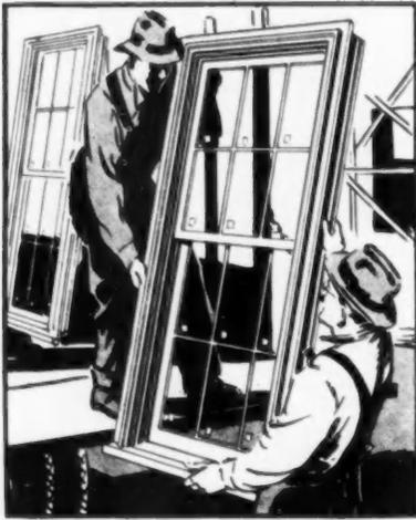
UNITS are delivered complete—frames are assembled, hung with precision-built, factory fitted, glazed sash, complete with weatherstrip and operating equipment.
