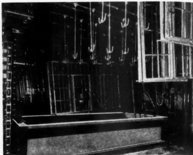
STEEL windows ("Fenestra") on moving hooks are dipped in a series of preservative baths in the Bonderizing treatment.
