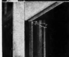
In the same manner as the upper sash, the lower sash is slide-sealed to the parting stop with special interlocking metal strips. Sash slide smoothly and easily insuring effortless operation.
