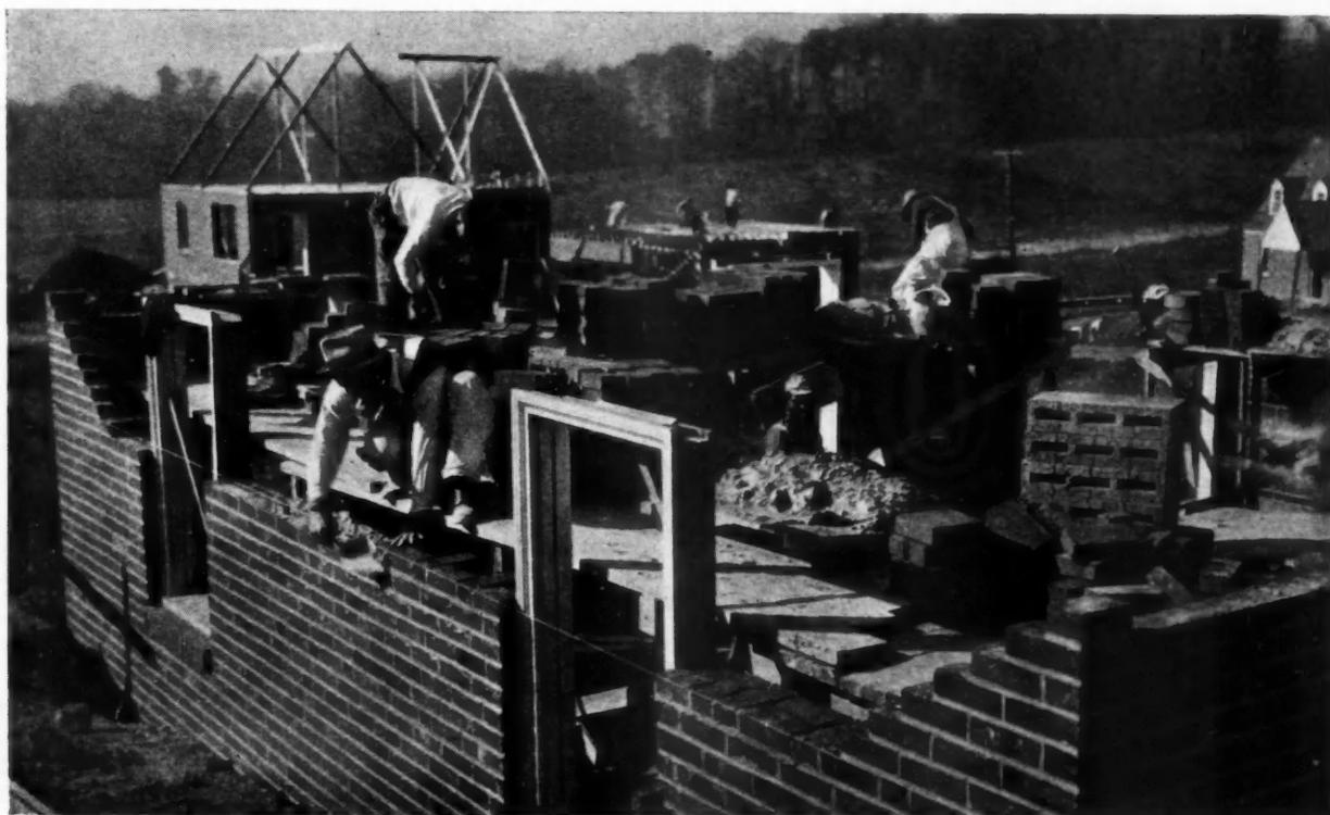
**MASONRY WALLS** of brick and lightweight concrete blocks (16" x 8" x 4") are used in Wilmington houses as workers rush to catch up with advance sales.
