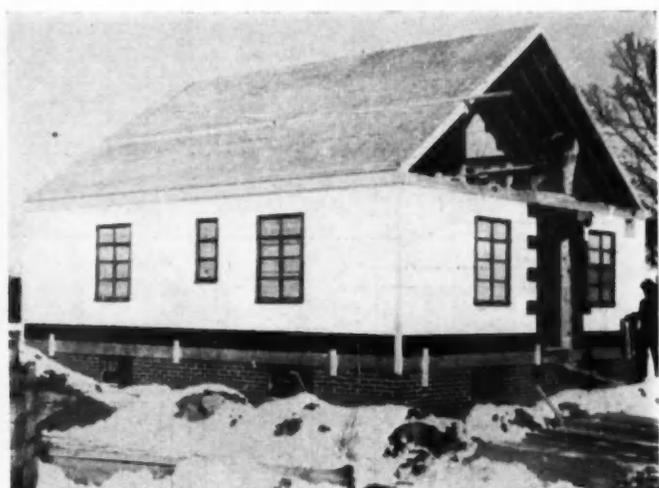
ABOVE: Foundation completed, wall sections are built on plywood subfloor; precut rafters and roof sheathing go up rapidly.
