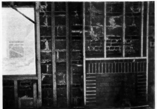
FURRING strips were nailed directly to 4" lightweight concrete blocks. Note tie-in brick course every second block.
