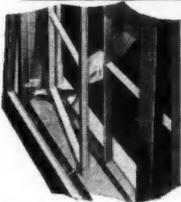
Linked to the casement ventilator at the sill, the storm sash opens automatically when the casement window is opened from the inside for fresh air.
