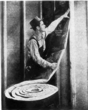
PLACING Red Top insulating blanket between studs.
