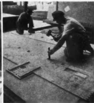
**WIRING** is inserted in wall sections at shop. **RIGHT**—Templates are used in cutting openings for outlet boxes.
