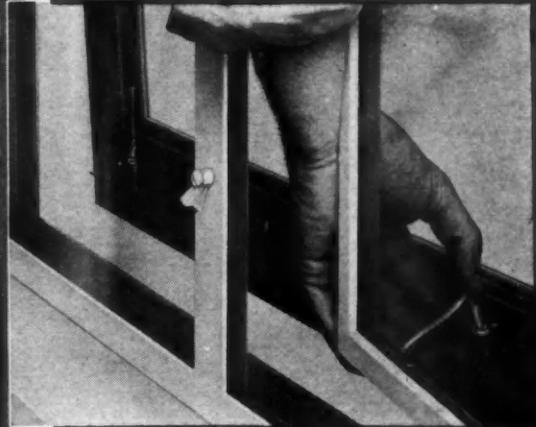
AT LEFT—As shown, you simply hang an ordinary storm sash at the top, on the outside of the Fenestra Package Window. Storm sash not supplied by Fenestra.
