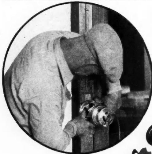
(Above) The Carter Templet mounted on the jamb, guides the Router for hinge recesses **SIX TIMES AS FAST!**
