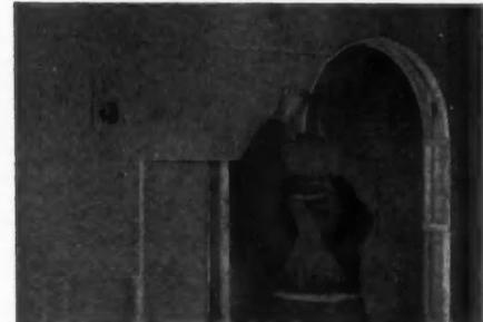
QUICK INSTALLATION is an important feature of Temlok De Luxe. Either adhesives or TEM-CLIPS can be used. Temlok replaces plaster and paint or wallpaper, hence avoiding the usual drying period.
