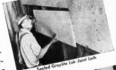
Sealed Graylite Lok-Joint Lath
