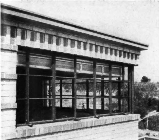
MODERN treatment of casement windows with vertical muntins omitted, and windows joined with mullions. This provides ventilation and daylight on the exposed corner of the building, as well as adding considerably to the modern appearance.
