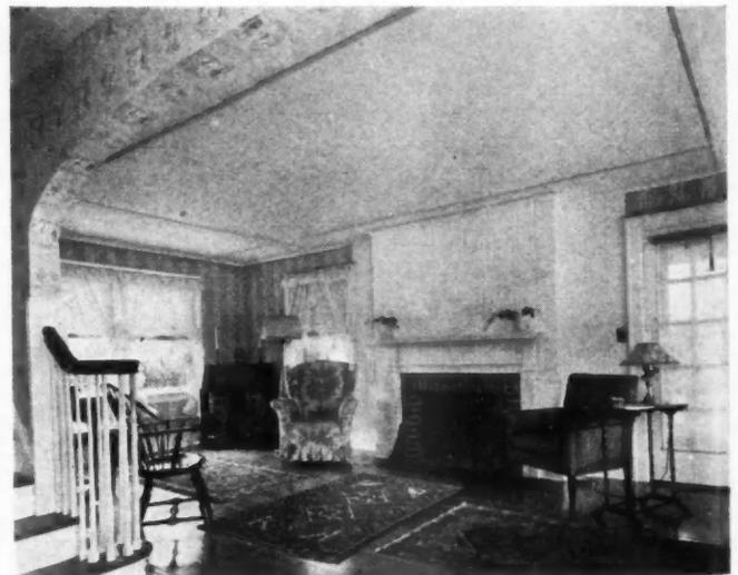
SOMETIMES it is possible to use a giant 8' x 14' Strong-Bilt Panel for the center of a large ceiling with a narrow border around it.
