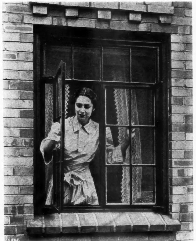
**EASE OF MAINTENANCE:** This photograph illustrates how double casement ventilators can be easily washed and cleaned from the inside of the house. Note also that the window is dropped one light, which makes it possible to install awnings, shutters, and other window fixtures without inconvenience.
