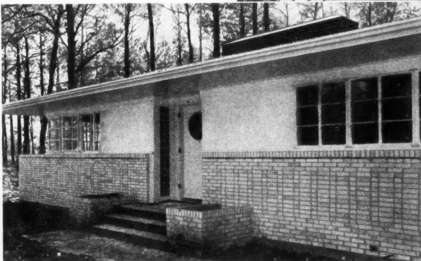
THIS Houston, Tex., home (plans shown in December '41 American Builder) has two Insulux block panels flanking the recessed entrance way. Here, light is the only consideration, and due to insulation value, fuel is saved. Below, a block panel lights the stairway in another Southern home.
