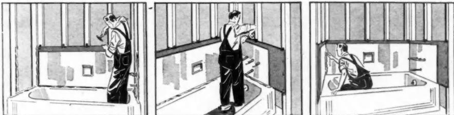
1. After buttering tub rim and studs with mastic, set the back plate of Carrara first. Nail through plasterboard flange
