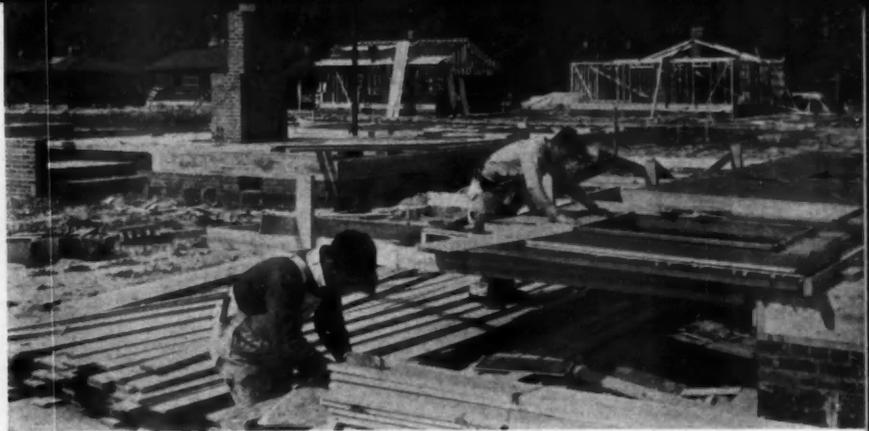
**APPLYING SIDING** to exterior wall in horizontal position. Doors and windows are installed and wall is completed before raising.
