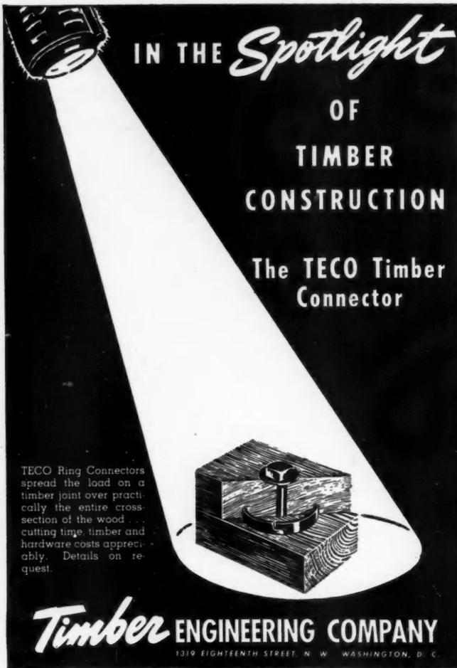
TECO Ring Connectors spread the load on a timber joint over practically the entire cross-section of the wood, cutting time, timber and hardware costs appreciably. Details on request.
