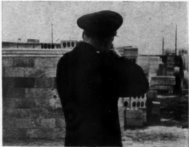
POLICE official is firing with rifle at concrete masonry wall in test at Franklin Park, Illinois.
