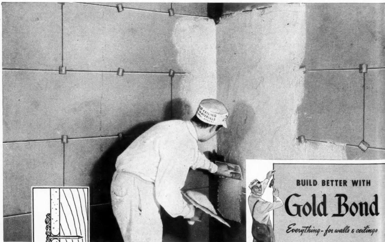
**NO SPECIAL EQUIPMENT IS NECESSARY** to install the Gold Bond Floating Wall System. Any lather can drive the patented nails *between* panels of gypsum lath, providing a resilient tie with the stud as shown in this diagram. Plastering is done in the usual manner.
