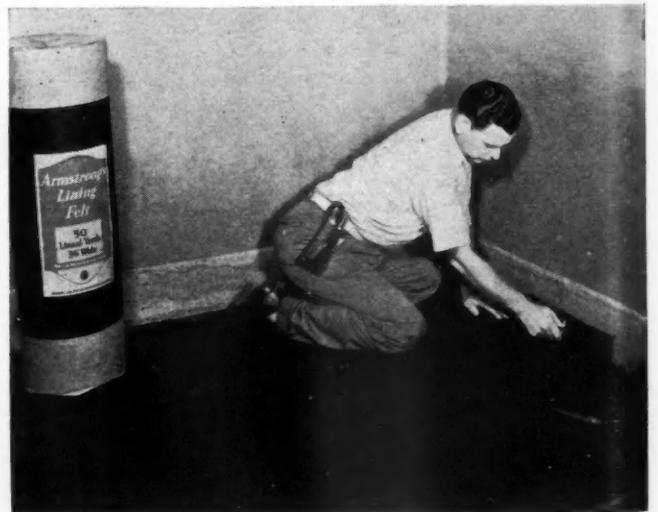
HERE a mechanic is applying Armstrong's new semi-saturated lining felt to be followed by linoleum.
