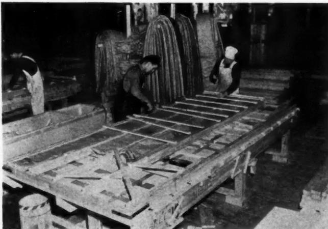
JIG TABLE used in building ceiling sections. Half-inch blanket-type insulation installed with tacker.
