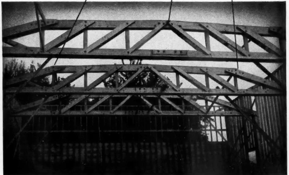
The use of 200 Teco Connectors releases more than a ton of steel, enough for approximately 400 army rifles, or 50 heavy machine guns.
