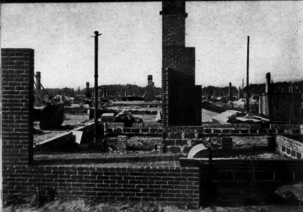
A FOREST OF CHIMNEYS rises from the site of the Levitt job as more than 300 foundations are completed before carpenters come on the job. Rough plumbing was installed first.
