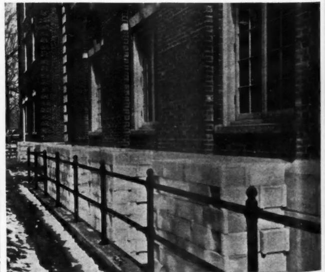
HOLLOW 12-in. concrete masonry units laid up without mortar are used to protect basement windows in dormitory building at Radcliff College, Cambridge, Mass., prepared for use as a bomb shelter.
