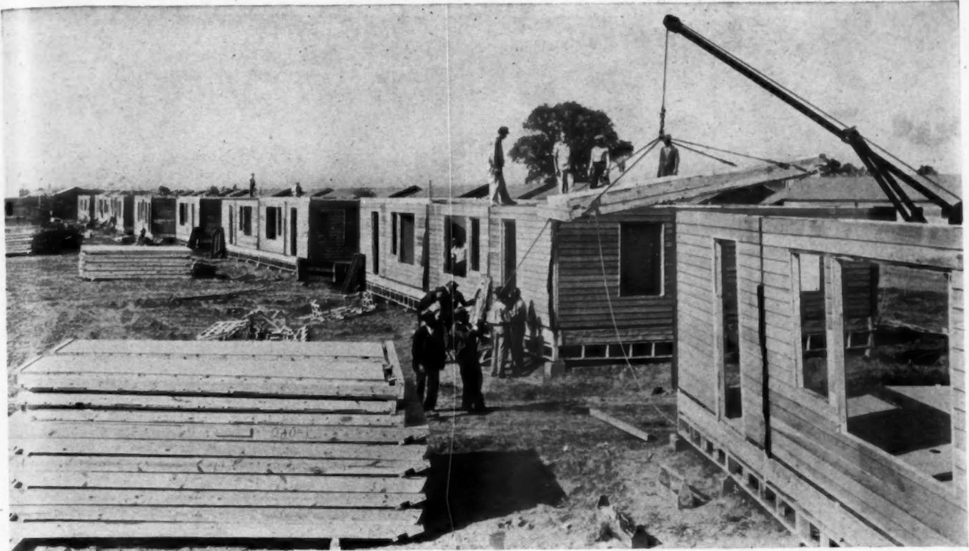
**CEILING SECTIONS** on long row of prefabricated demountable units are lifted into place with truck-mounted boom.
