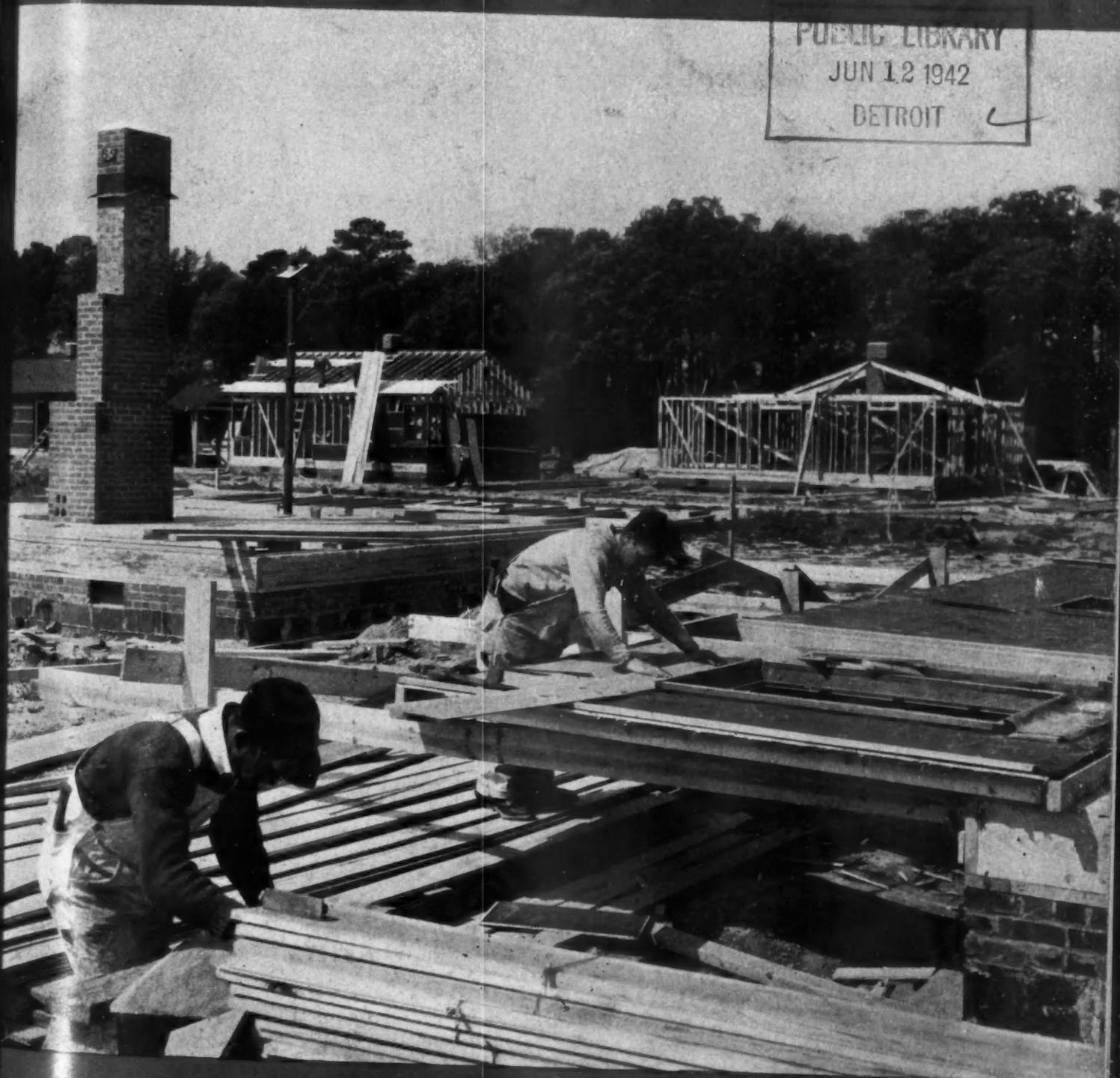
Levitt workmen speed this war-housing job at Norfolk by applying siding to walls lying flat.
