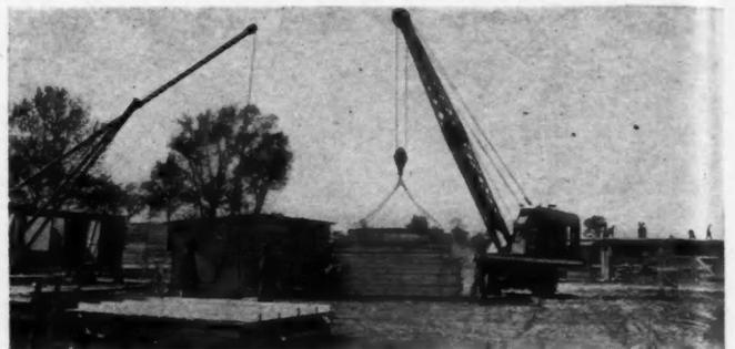
**HEAVY CRANE** transfers prefab sections from truck to site.
