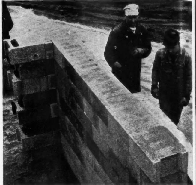
WORKMEN are inspecting concrete masonry wall after test with high velocity rifle fire at Franklin Park, Illinois.
