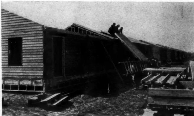
**LABORERS** slide roof sections into place on long row of demountable units.
