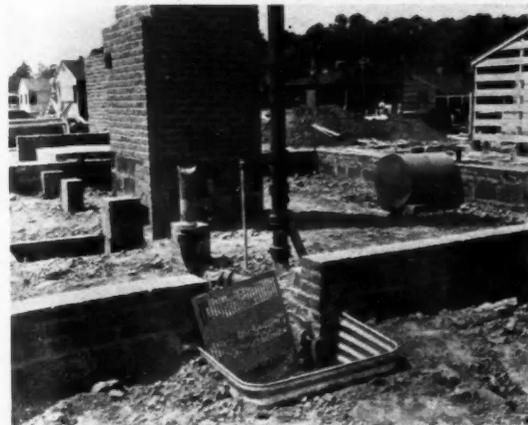
**COMPLETE FOUNDATION** with metal areaway, rough plumbing and oil tank; concrete pit for floor furnace.
