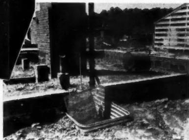
Typical Levitt "All American" Home under construction at 200-acre Oakdale Farms, Norfolk, Va. Pit for International Floor Furnace at left; oil tank at right.
