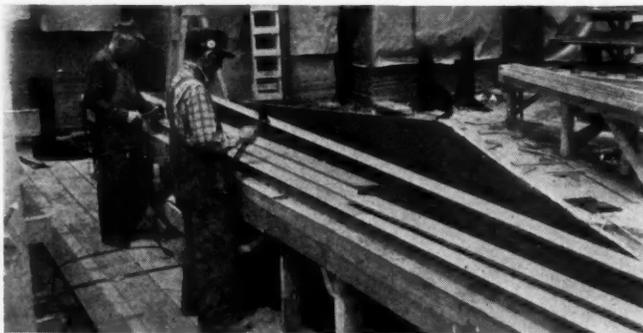
BUILDING END GABLES on special jig table. Redwood siding is nailed direct to 2 x 3 studs covered by 30-lb. felt.
