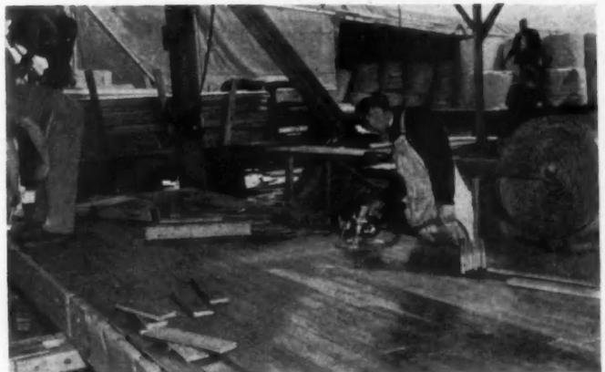
**AT FACTORY,** floor sections are built two at a time, cut apart by power saw. Units are insulated with ½" blanket, have factory-finished oak floor surface.
