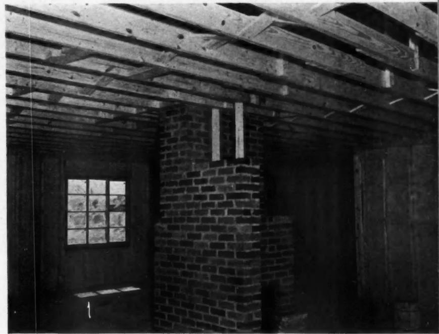
**CEILING HUNG** from roof rafters so that interior finish can be applied without fitting around partitions. These are installed *after* gypsum board has been applied to entire ceiling and interior plywood finish to outer walls.
