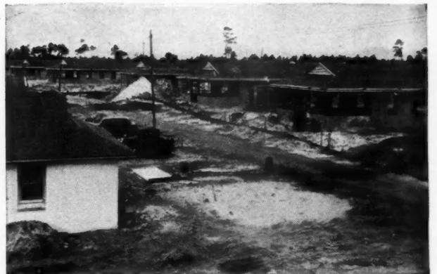
● Army Hospital Area under construction at U. S. Army Base. Stucco made with Atlas Waterproofed White cement was applied over hollow tile.
