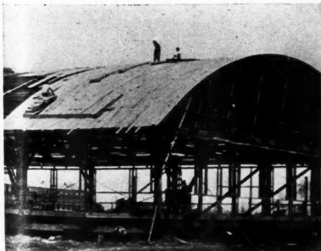
**SAVING STEEL—**Men on the job sheathing over 166-foot clear span trusses constructed of wood reinforced with timber connectors. Mold loft buildings such as the one above have been duplicated many times in shipyards on the Pacific, Atlantic and Gulf Coasts. Unobstructed floor is giant drawing board. (OWI Photo.)
