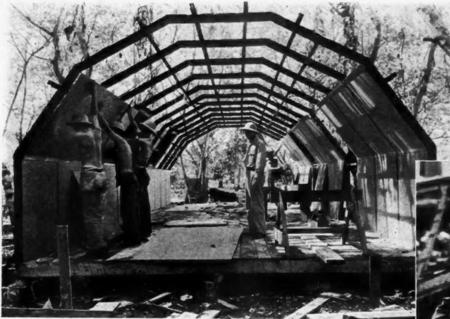
**SOMEWHERE IN THE SOUTH PACIFIC**—These Navy Seabees are stripped for action and hard at work putting up a Quonset Hut in a jungle clearing. The Seabees are composed of bluejackets and officers who construct camps and bases at advanced points. They also erect barracks, airfields, docks, gun emplacements, etc. (Official U. S. Navy Photographs.)
