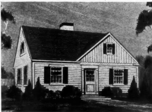
ABOVE: Sketch of story-and-a-half war housing unit built by Gerholz-Healy, Flint, Mich. WPB allows attic area having 5 feet or more clear head room to be added to first floor area in figuring total in this design.
