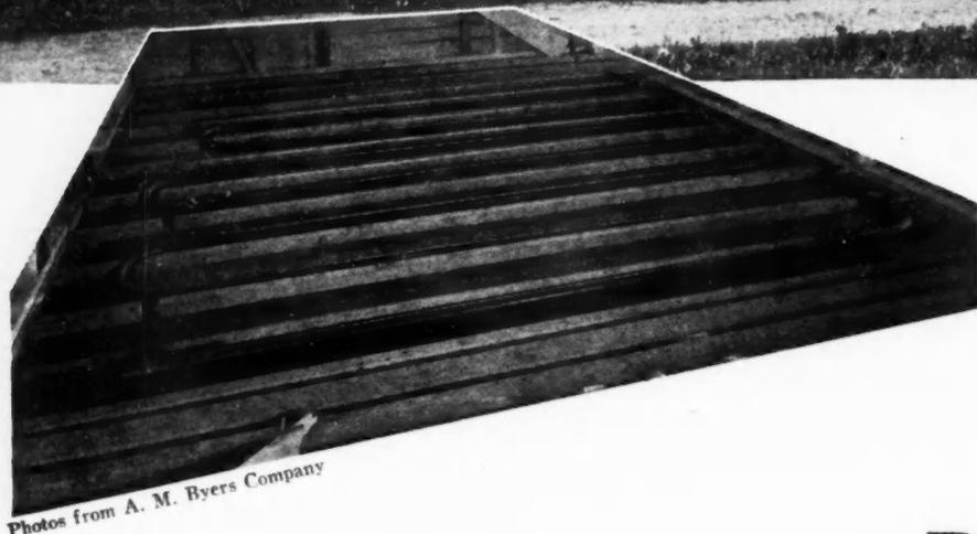
**THAT HUGGING-the-ground appearance adds to the architectural charm of a house. Radiant heating permits this by making the basementless house more practical than ever. The owner of this home wanted hardwood floors. Picture at left shows how this was accomplished. The coils rest on a concrete slab, and the hardwood floor is laid on sleepers notched to receive the pipes.**
