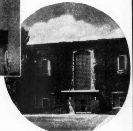
**In Factories**—Panels of Insulux can help the manufacturer solve many problems of light, temperature, humidity and dust control.
