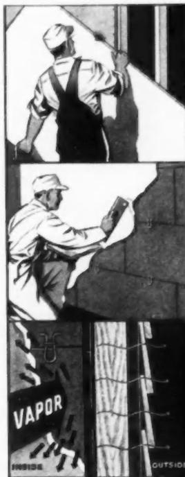
**OUTSIDE THE STUDS,** Insulite Bildrite Sheathing. The large boards provide a wind-proofed, weather-tight wall. Bildrite Sheathing has a bracing strength four times that of wood sheathing, horizontally applied.
