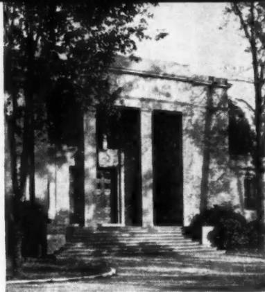
A successful combination of concrete units and cast stone trim is seen in this entrance to the Drill Hall. All masonry units were made with Lehigh Early Strength Cement.
