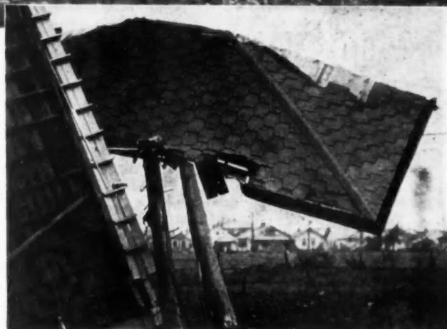
Roof deck blown completely off, but with practically every Cyclone shingle intact.
