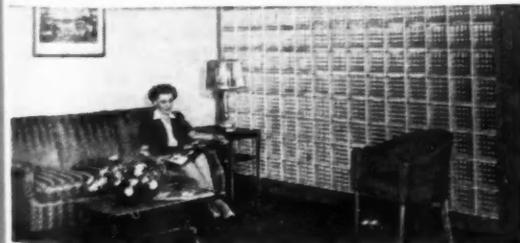
It is easy to change the size of any room with an Insulux partition. Furthermore—the edges of the wood strips may be painted so that the panel harmonizes with the decorative scheme.
