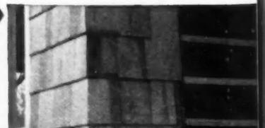
**BRICK**—Wall ties for masonry veneer shall be nailed securely through the sheathing to the wood framing. Air space of 1" shall be left between sheathing and back of veneer.
