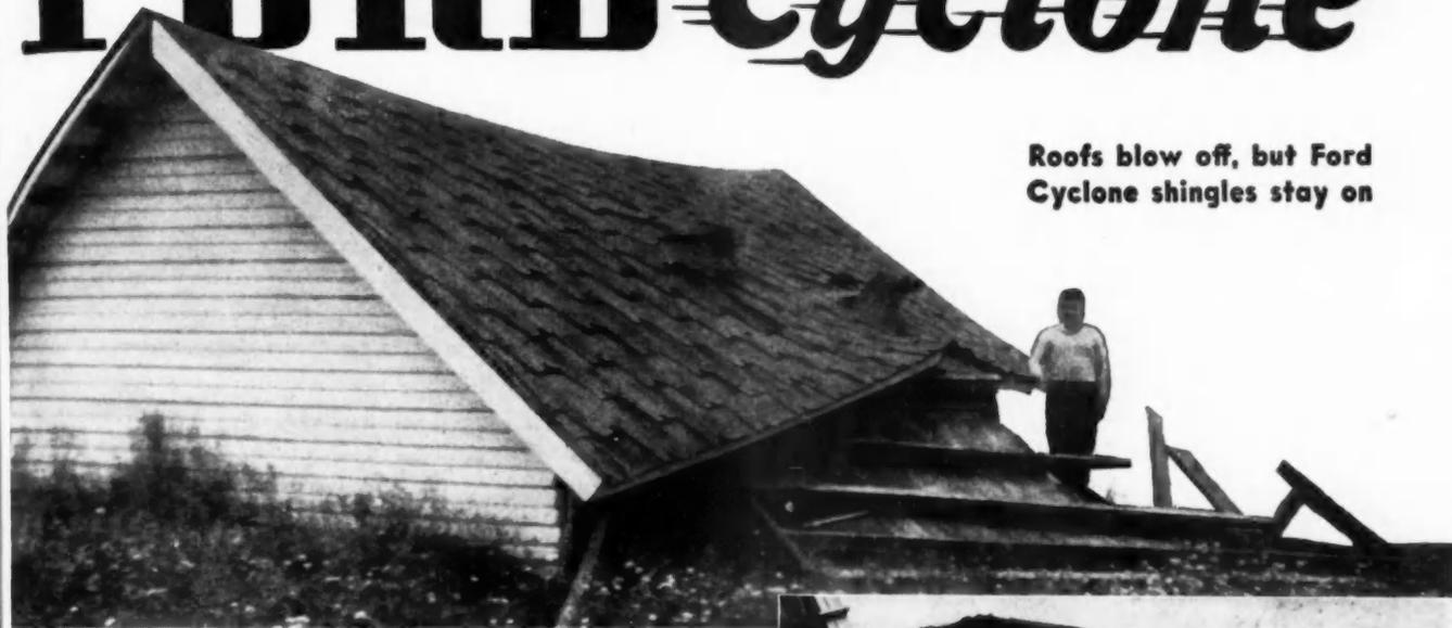
This roof was carried 40 feet, with no damage to the Cyclone shingles except that caused by the 2 x 4 studs pushed through the roof.
