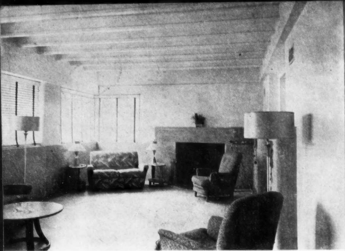
LIVING ROOM of Haddonfield, N.J., home showing exposed Lith-I-Bar joist ceiling, eliminating the cost of ceilings and providing an excellent acoustical effect. All first floor level floors have 1 inch of terrazzo finish on a 2½-inch concrete slab poured on Lith-I-Bar joist, providing an attractive, permanent type of floor.
