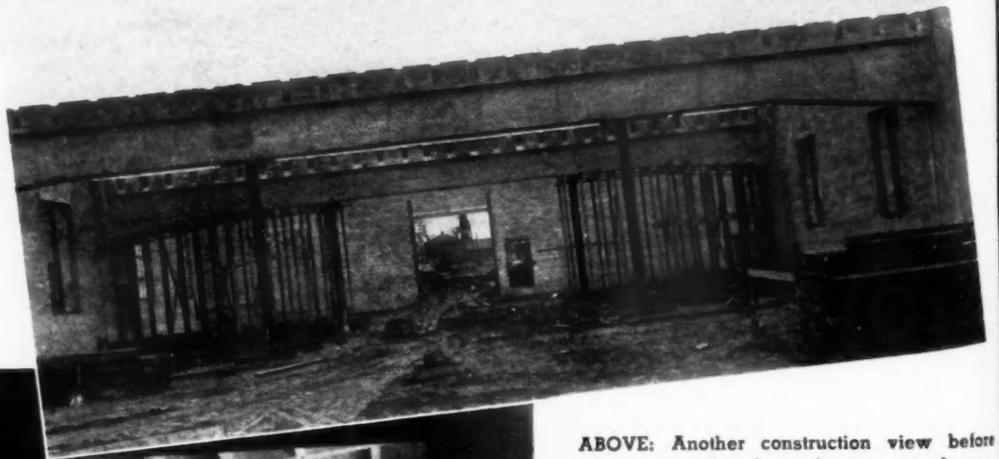
ABOVE: Another construction view before joists were placed on the concrete beams.
