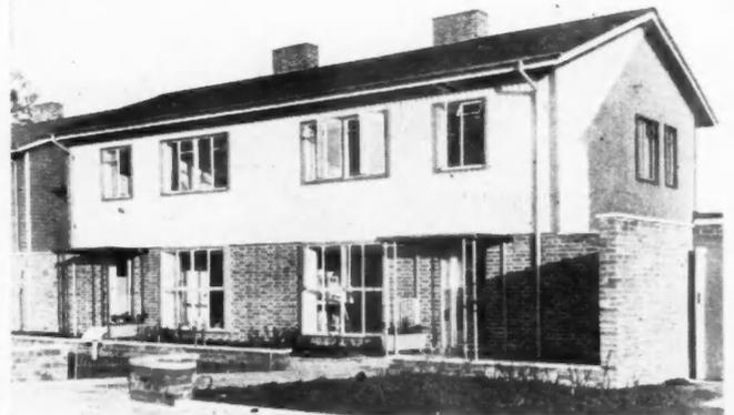
ONE of Britain's new steel and concrete houses, designed by the British Iron and Steel Federation, is shown above.
