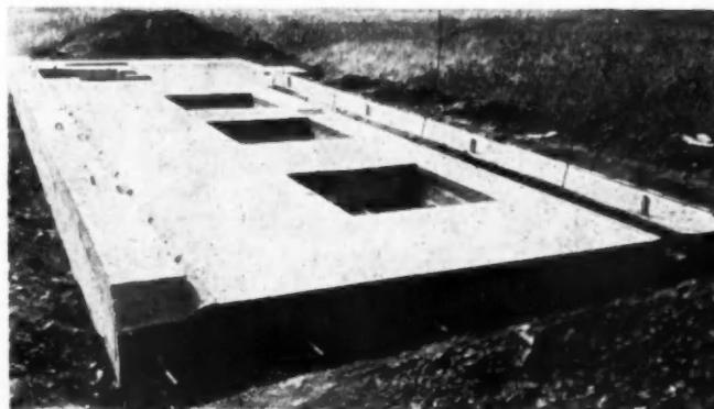
COMPLETE wall unit, including fireplace, ready to erect (tilt up). The foundation and the two walls are separated by air space.
