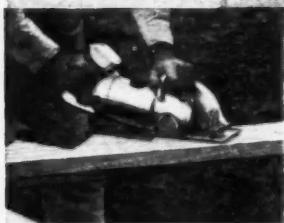
**CUTTING STAIR STRINGERS** with a B & D Electric Quick-Saw finishes the job in a fraction of the time required by hand.
