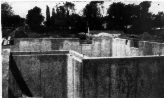
Smooth-surfaced, straight walls of uniform thickness—accurate inside and outside corners are assured on every UNI-FORM foundation. Boxing out and brick ledges are very easily handled.
