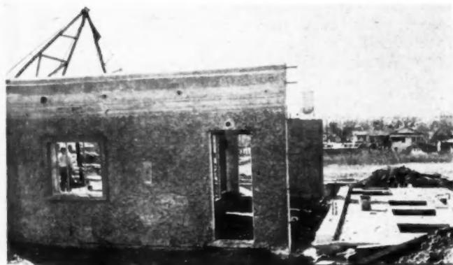
WALLS being lifted. Cast on the ground, they are in their proper place on being tilted up. Welded steel rods fasten the corners.
