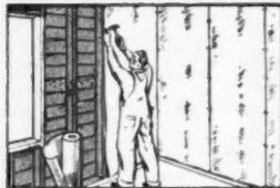
Using Sisalation means that both insulation and moisture vapor barrier can be installed at one low material and labor cost.
