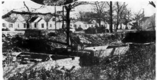
THIS small model track-type tractor can excavate two basements a day.
