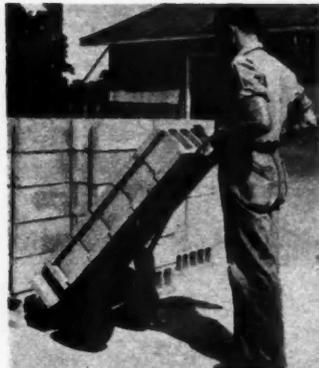
AB28161—The Reed Block-Man, a product of the R. S. Reed Corp., Three Rivers, Mich., is a hand truck with forks which enables one man to pick up and transport six concrete blocks at one time. The bottom block on each pile is laid face down and thereafter serves as a pallet. The loaded truck will roll freely over soft ground.
