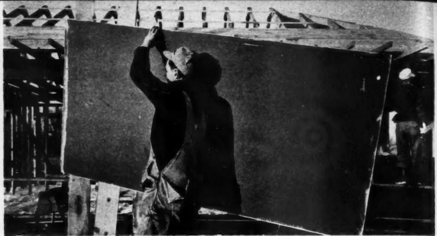
**KIMPREG-PLYWOOD** panel ready for installation in wall is handled by one workman
