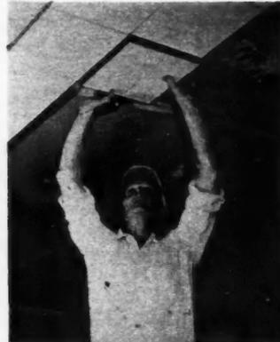
AB28155—A light-weight, low-cost acoustical tile with high sound-absorbing properties for ceilings is announced by Owens-Corning Fiberglas Corp. Painted white at the factory, the tile has a felted fiber surface and is beveled on all four edges. It can be cemented to a solid backing, or it can be mechanically mounted on wood.
