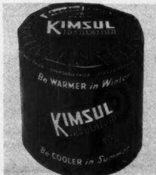
AB28172—A notable improvement in Kimberly-Clark Corp.'s Kimsul insulation during 1947 was introduction of the use of Pyrogard fire-resistant cover paper. The three thicknesses of Kimsul building insulation—standard, commercial and double thick—shipped in the familiar compressed roll, are all now covered with this new paper.
