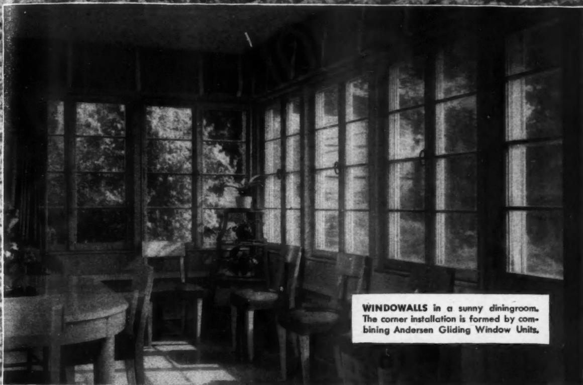
**WINDOWALLS** in a sunny diningroom. The corner installation is formed by combining Andersen Gliding Window Units.
