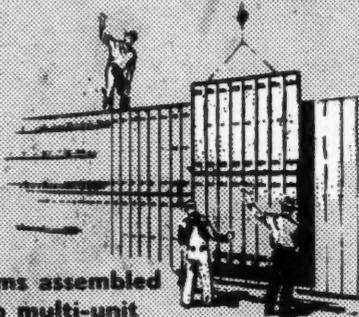
Forms assembled into multi-unit panels for rapid crane handling.
