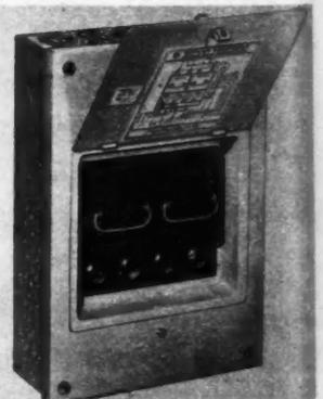
AB28176—The Frank Adam Electric Co., St. Louis, Mo., announce a new main and range electrical service unit. It is designed to meet modern requirements for homes equipped with electric ranges or other heavy capacity appliances. Box has ample wiring gutters, keyhole type mounting slots, 21 knock-outs and well-located terminals.
