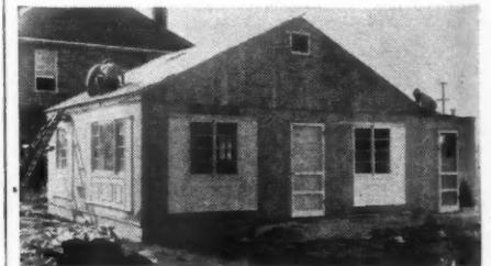
**ROOFERS** putting finishing touches on factory-built house held intact with glue
