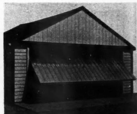
AB28229—The Berry Door Co., Wayne, Mich., has added a new single span double door to its line of aluminum garage doors. Light and perfectly balanced, the 16x7-foot door tilts up and rolls completely into the garage, smoothly and quietly. Heavy bracing assures rigidity and a new type of face grooving gives this new door a smoother, more distinctive appearance in addition to greater strength. Shipping weight, crated, 170 pounds.
