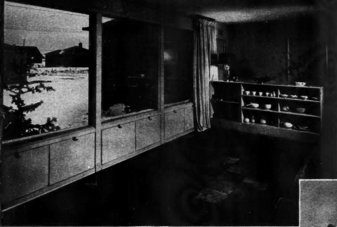
**HASCO block flooring** in place in living room. Blocks were laid directly on concrete with mastic. Note pleasing pattern resulting from red oak grain in blocks. Below, laying flooring on cement slab with mastic
