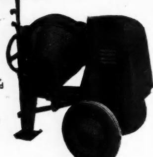
Welded steel drum locks in any position
