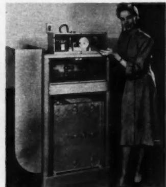
**AB28228**—The Trion electric air filter made by Trion, Inc., McKees Rocks, Pa., utilizes electrostatic precipitation for removal of foreign particles from air streams. Photo shows inner workings with panel removed and power pack taken out of position and placed on top of unit. Made in several sizes for homes and commercial buildings.
