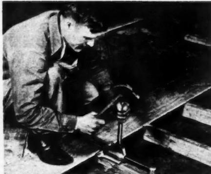
**AB28126**—Here is a tool designed for quick application of flooring, siding and sheathing with the tightest possible joints. Patterned on a lever principle, similar to a jack, it can force even badly warped boards into line and hold them in position for nailing. A tap of the hammer against anchor sets tool into position on joists, and lever action squeezes the boards together. The tool is made by Maco Corp., Huntington, Ind.
