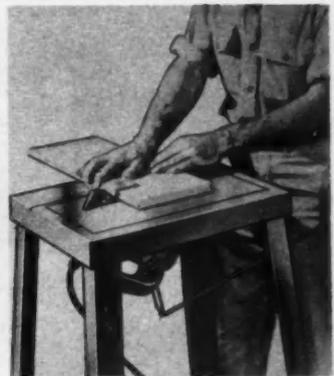
**AB28166**—The Model 60 MailSaw is a sturdy, portable electric hand saw weighing only 8 1/2 pounds, and is manufactured by the Mail Tool Co., Chicago, Ill. With the available saw table and attachments, the Model 60 may be used for sanding, grinding, wire brushing, sharpening tools and knives, drum sanding, and other jobs.
