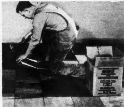
AB28232—Hasco block flooring is a prefabricated, pre-finished flooring of balanced construction that has little or no expansion or contraction. Product of the Haskelite Manufacturing Co., Grand Rapids, Mich., it can be laid in mastic right on a concrete sub floor or laid in any modern home. The 12-inch by 12-inch size fits architectural specifications and achieves a pattern of pleasing appearance. Red Oak is the material used for construction.
