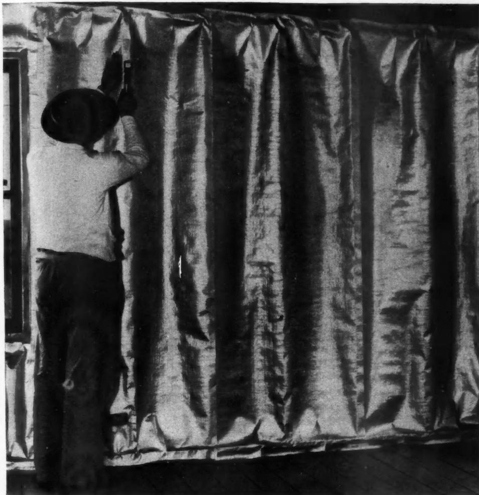
**1** You get insulation that is completely effective, since SISALATION, properly applied, is equivalent in heat-saving values to approximately  $\frac{3}{4}$ " of flexible or rigid types of good insulations most commonly used...based on M.I.T. tests on sidewalls constructed with a single layer of reflective SISALATION.
