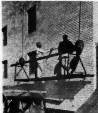
**AB28111**—Safway Steel Products, Inc. of Milwaukee makes this light duty swing stage, called Saf-T-Swing. It is designed especially for such jobs as maintenance work, painting, cleaning, tuck-pointing, etc. The new winch design increases safety. Two winches, entirely gear-operated, are each equipped with 150 feet of steel cable.
