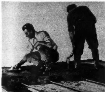
AB28209—Zonolite Stabilized Concrete Aggregate is becoming increasingly popular to produce insulating concrete floors. When placed beneath radiant heat ducts or coils, Zonolite concrete prevents wasteful heat loss into the ground and facilitates efficient and economical operation of the heating system. These floors have been widely used in rural, commercial, industrial and residential building, with or without radiant heating systems.
