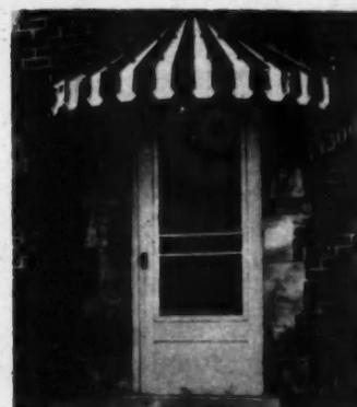
AB2805—This circular aluminum doorway canopy, made by Koolvent Aluminum Awning Distributors, Inc. of Pittsburgh, has smart styling and color, and is installed easily. All-weather protection keeps doorways free of ice, snow and rain, and prevents warping of doors. Vents and louvers let air through, but reduce and diffuse light.
