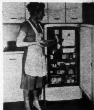
AB2832—Two additional cubic feet of refrigerated storage space is made available in the new line of General Electric refrigerators. Leader of the line is an 8-foot box that takes the same floor space used by the former 6-foot box. The extra refrigerated space is made possible by development of a smaller refrigerating unit.
