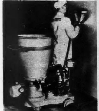
AB2846—Colorcreting is a process of pneumatically applying a cementitious material to exterior and interior masonry surfaces. Colorcreting outfit consists of a mixing drill, compressor, electric or gasoline motor, a length of hose and a gun. Outfit and materials are available from Colorcrete Industries, Holland, Mich.
