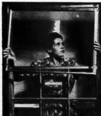
AB28191—The Aluminum Window Corp., Garden City, N.Y., announce a new type storm window and a new type screen, both of the roll type, which can be installed on all kinds of windows. They also reveal improvements in their Alwintite double-hung windows to reduce air infiltration. Windows are assembled at factory.
