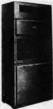
AB28160—Frigidaire is now producing a five-ton capacity packaged air conditioner, especially designed for stores, restaurants and business houses. Occupying only 7 1/2 square feet of floor space, the new unit is completely self-contained. The refrigerating unit, electric motors, cooling coils and fans are all housed in one single cabinet.
