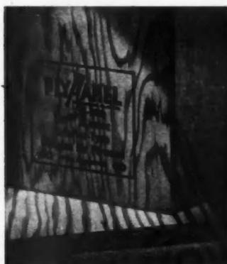
AB2871—This unretouched photo of Douglas fir plywood panels show clearly two of the industry grade trademarks for ready identification of types and grades of fir plywood. Upright is Plypanel Sound I Side grade interior type for use where one side is to be exposed. Horizontal is same grade exterior for use on outside sidewalls.
