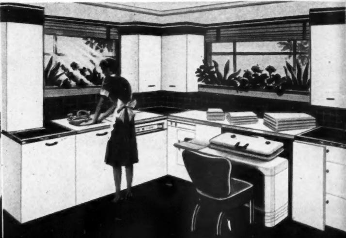
The Automatic Laundry has an automatic washer, automatic clothes dryer, and flatplate ironer. Here electricity does all the drudgery out of washday.
