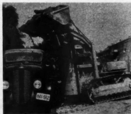
AB28111—The Caterpillar Tractor Company's diesel D4 track-type tractor, equipped with Traxcavator, is utilized by builders to excavate foundations for houses and other structures at the start of construction work. When construction is actually under way, the unit is suited to numerous jobs on the site, especially for back-filling and leveling ground. This tractor is one of a number of units which are manufactured by Caterpillar Co. for use by builders.
