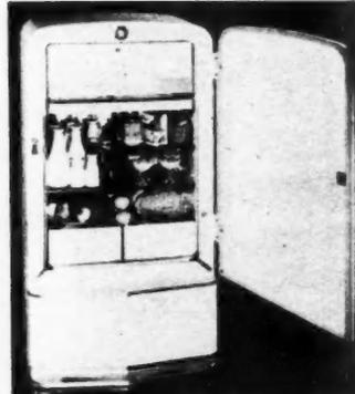
AB2864—The new seven cubic foot Westinghouse two-temperature electric refrigerator shown above will hold 56 pounds of frozen food, 43 in the freeze chest and 13 in the ice storage compartment. The temperature selector controls the temperature of the freeze chest, while the second control governs the general food storage area.
