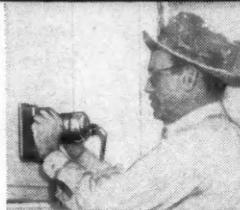
EASY cuts no swirls or other abrasive marks. Straight-line action produces "hand sanding" results on white wood, filler and final coats in 1/3 the time. For CURVED or flat, WET or dry work. EASY is not a disc, belt or orbital sander.
