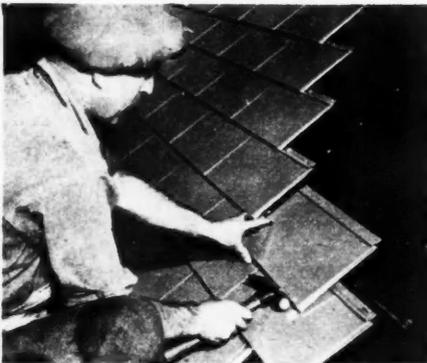
AB28113—Rustproof, fireproof, rotproof, Reynolds Lifetime Aluminum shingles eliminate maintenance. Their surface is raised away from the sheathing of the roof, providing an air space faced by aluminum, which reflects as high as 95 per cent of radiant heat from either direction. Easy to apply, because they are self-aligning, they can be painted or left unpainted, in which case, natural weathering tones down brightness.
