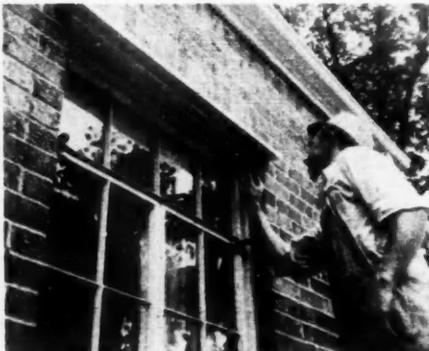
AB28105—The Aluminum Building Products Co., East McKeesport, Pa., announce the "Lewshield" window and door cap, rigidly made of aluminum alloy in a neat and pleasing ornamental design. The item is made in two widths—4 inches for small openings and 5½ inches for larger openings. Both are available in standard sizes or may be obtained in any special length up to and including 21 feet, adaptable for all different styles and types of windows.
