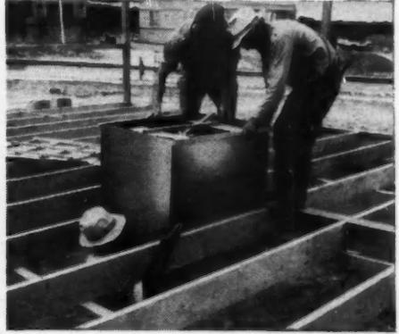
**Easy, economical installation.** This photo shows a Coleman Floor Furnace in place—in the floor, not on it and not in the basement. No basement is needed, so often you can save the cost of excavation; and you save much costly duct work. Easy to connect with chimney and fuel line. Models from 25,000 to 70,000 BTU input or equivalent; single or multiple installations.
