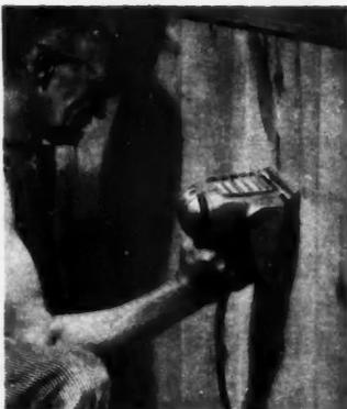
AB2844—The new model Sterling 1000 Portable Electric Sander to be introduced at the Chicago show, has three new features. An air scoop protects it in extremely dusty operations. Side housing fenders protect transmission. An auxiliary handle gives added support for vertical and overhead work. Made by Sterling Tool Products Co.
