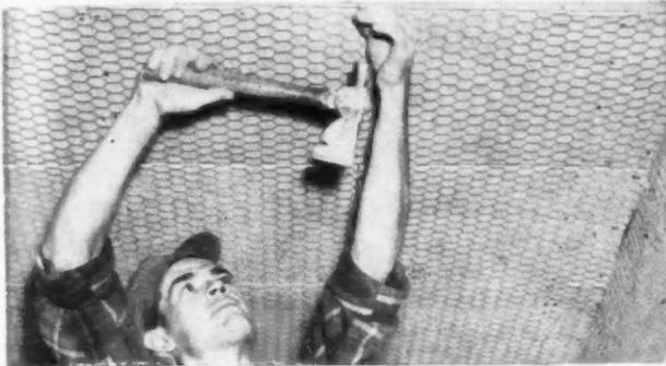
Lathers applying Keymesh Reinforcing to ceiling. Notice how the reinforcing protects the ceiling-wall juncture.
