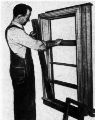
that can be used with any type sash balance. Allows warped sashes to slide freely and easily with weather tight protection. Can be used on either rabbeted or unrabbeted jambs. Department AB, Macklanburg-Duncan Co., Oklahoma City, Okla.
