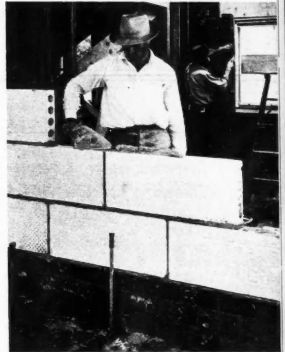
GYPSUM block, brick and similar materials are used with concrete slabs
