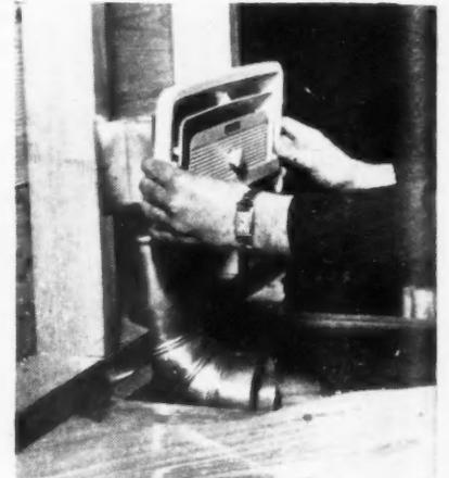
**FITTING** register to register box on cut-away model of typical home installation stated. Air is supplied at somewhat higher temperatures for mixing with room air as it leaves the registers. (Continued on page 212)
