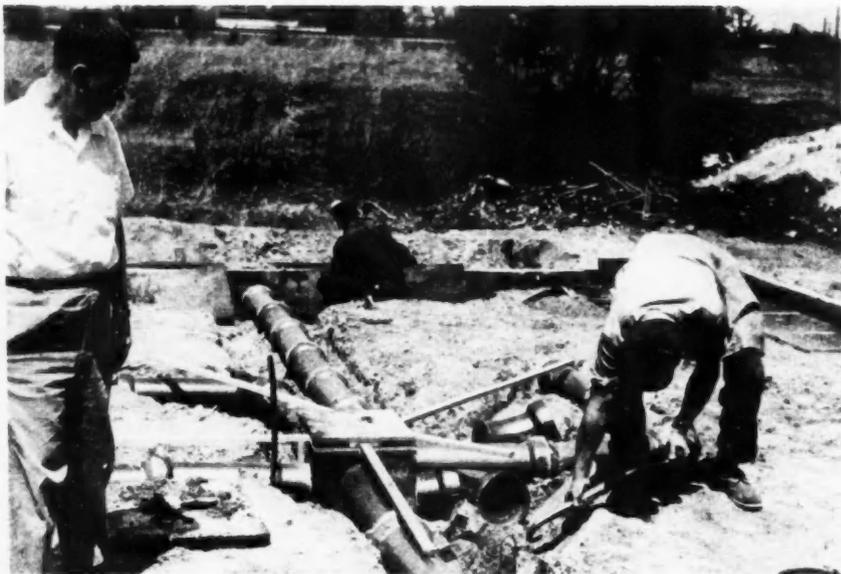
INVERTED blower type oil-fired furnace supplies heat through clay pipe ducts to warm air registers in rooms. Heat loss is exceptionally small, according to Virgil Place
