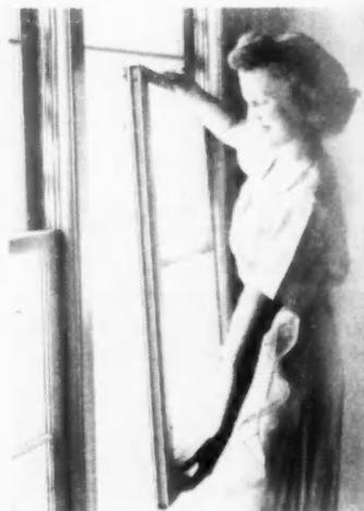
both sash. Parting stop is part of the vertical rail. Pressure for holding the sash in desired position is obtained by two continuous rubber strips, functioning as springs, placed on back of vertical rail opposite stiles of sash. Named "Seal-Rite," this weather strip provides draft-tight windows. Seal-Rite Manufacturing Co., 600 Michigan Building, Detroit 26, Mich.
