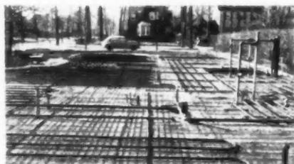
*B & G Hydro-Flo Radiant Panel installation with pipe coils in concrete floor.*
