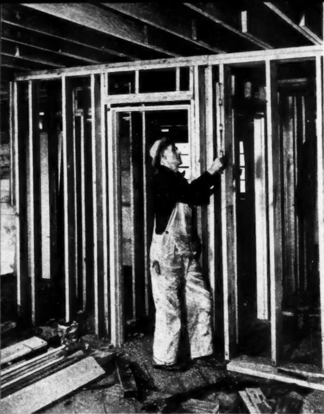
AN example of a typical wood stud bearing partition in a frame house. This is a type most frequently used
