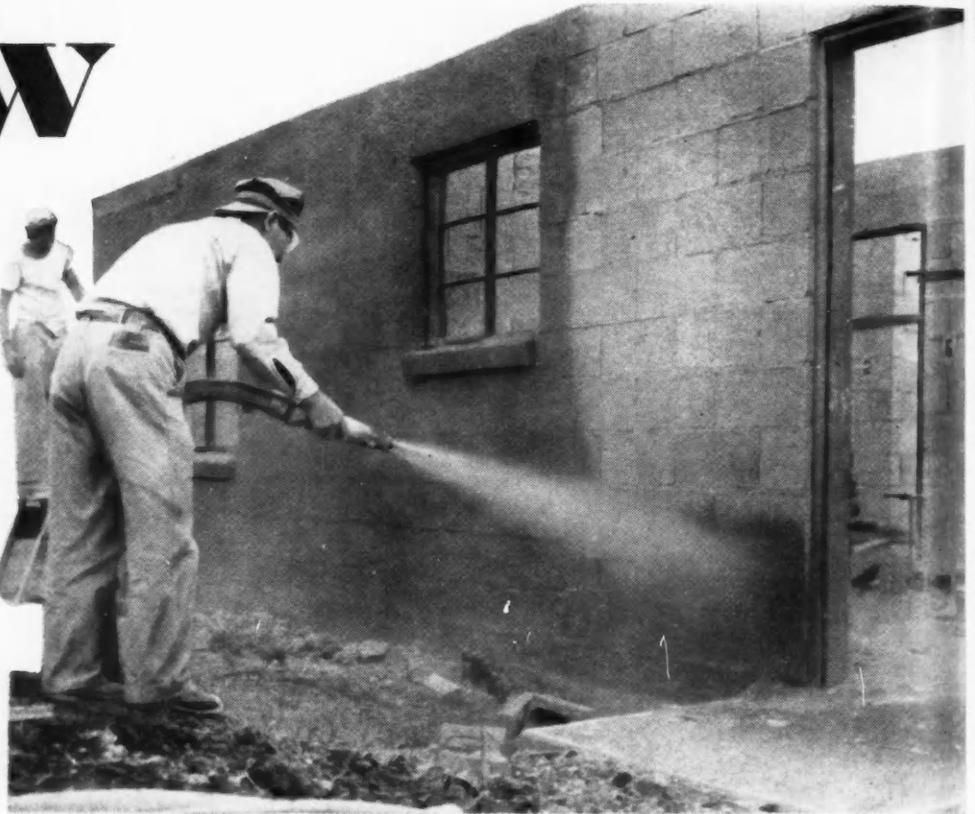
**T**WO hundred and eight of these FHA-approved concrete masonry homes, with 640 sq. ft. of floor area, have been recently built in Fort Worth, Texas, by the Farmer Construction Co., Inc., of that city. Foundation slabs were placed with Lone Star Cement concrete. Next, haydite light-weight-aggregate masonry units were laid up. Then a 1:3 Lone Star Masonry Cement—sand mortar exterior coat, approximately three-quarters of an inch thick, was applied with Jet-crete gun in about one hour's time.
