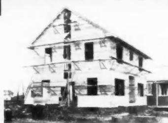
Builders and contractors are quick to see the time and money-saving advantages of "Trouble Saver" Equipment... and the extra safety provided. Use of "Trouble Saver" Scaffold brackets and ladder jacks speeds work and eliminates many working hazards that cause costly accidents. Safe working platforms help your men do more and better work.
