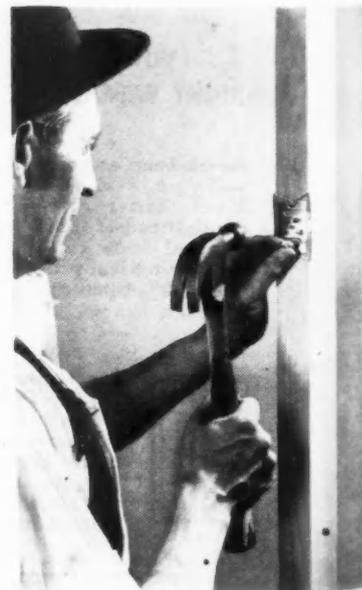
*It is so simple! Nail Fasteners to studs in new construction. Fastener prongs enter back of panel and clinch.*
