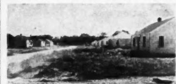
**THIS WAS TAYLOR STREET** in the Seaman Gardens subdivision after the flood waters had receded. Most of these homes were covered with asphalt-cement shingles over gypsum sheathing. Shingles and sheathing performed well under the flood battering
