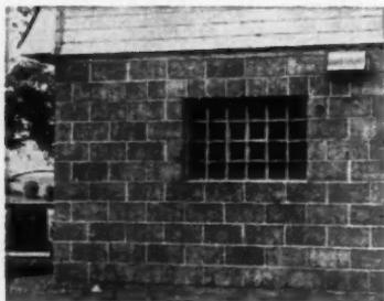
**TWO glass block designs** were used here in combination, the clear block allowing vision with no loss of insulating quality
