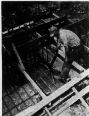
A pneumatic concrete vibrator designed to compact freshly poured concrete and to direct its movement as it is poured into the form, is called the Thor No. 521 Vibrator and is made by Independent Pneumatic Tool Co., Dept. AB., Sales Promotion Div., 175 N. State St., Aurora, Ill. Unit consists of 2 1/4-inch diameter steel cylinder, 17 1/2 inches long at the end of a five foot combination air and exhaust hose. Rotary air motor and vibrator unit are sealed in the steel cylinder.
