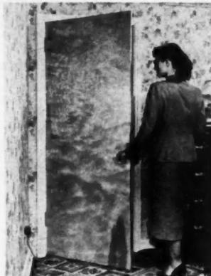
A seven-ply construction plywood flush door of birch and gum panels is the product of Walled Lake Door Co., Dept. AB., 1225-A E. West Maple, Walled Lake, Mich. The firm has also introduced the double lock block, which allows hardware installation from either side, rotating of doors for matching grain effect, and positive door balance. Of all-wood construction, the core frame contains about 9 1/2 square feet of lumber. The doors are easy to install and easy to finish.
