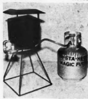
Designed for winter building is the new "Portable Heater". It delivers 40,000 B.T.U.'s and is capable of raising room temperatures 50 degrees in 20 minutes. The lightweight, 55 pound unit is easy to carry and its operational cost is estimated by the manufacturer to be \$1.00 a day. The heater is sold on a money-back guarantee, with a 30 day trial period. Manufactured by The Portable Heater Co., Dept. AB., Box 444, Painesville, Ohio.
