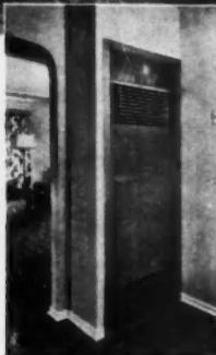
Back of unit also has cold-air-intake and warm-air-discharge grilles that provide circulated, uniform whole-house heating.
