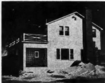
**PANELS** of glass block used to replace windows on sun porch of a farm home. Glass block were used also in openings on each side of the chimney
