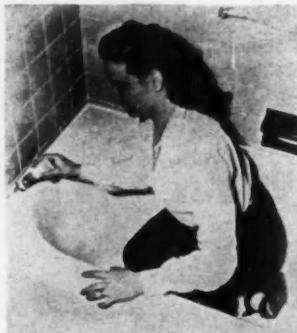
Caulking is neat, quick and permanent with a product that is applied like toothpaste and which dries in an hour leaving a tough, waterproof bond. Called Tub-Caulk, the product is designed for waterproofing around shower stalls, for caulking around bathtubs and sinks and for filling cracks between window frames and tile or plaster. Its finish is white and velvet smooth. The product is made by Miracle Adhesives Corp., Dept. AB., 214 E. 53rd St., New York 22, N. Y.
