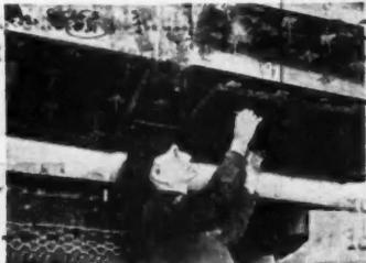
3. FIBERGLAS Insulation Type PF-613, 2" thick -- bonded to concrete ceiling using MIRACLE PRONGED ANCHORS at Radio City Studio 68, New York, N. Y. CONTRACTOR, William J. Scully, Inc., New York, N. Y.
