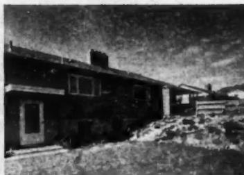
Partial view of rear elevation. Higher level at porch conforms to the street front. Rock garden planting covers the terrace between the two levels. Canopy over basement door is at floor level. Joists are extended to form the supporting members. Above grade windows supply ample light to basement area
