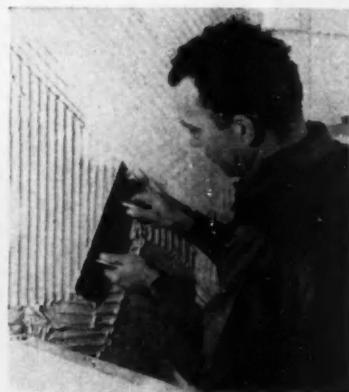
MASTIC is applied to the wall first in a vertical and then in diagonal pattern
