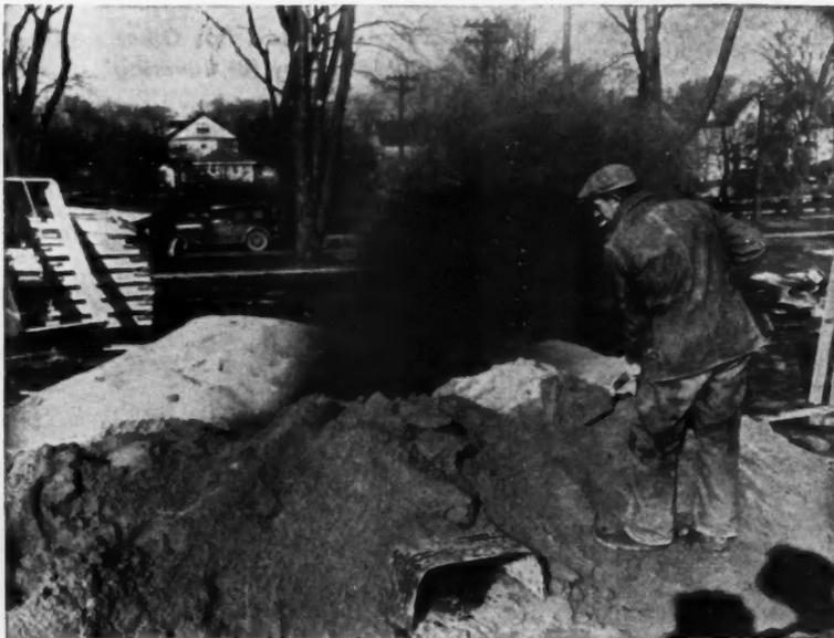
**SIMPLE METHOD** of heating sand and aggregates is to pile them over a 14 to 18-inch piece of culvert or heavy pipe and build a fire in the pipe. Setting the water barrel at one end of the pipe will heat water at the same time aggregate is being heated
