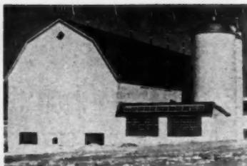
**GLASS BLOCK** on the farm serves dual purpose of light admittance plus insulation from frost and drafts
