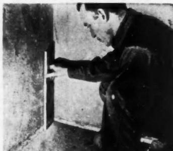
FIRST step is to measure for leveling point and to square and plumb all corners
