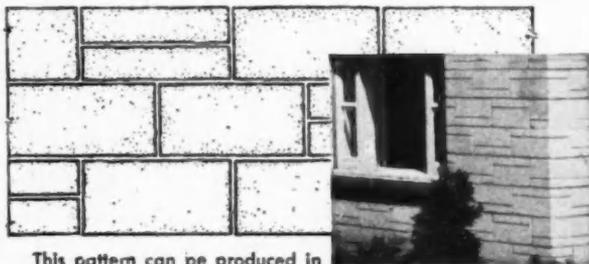
This pattern can be produced in many variations by using 8x8x16-in. block, some of which have been scored with a masonry saw. The finished wall appears to be made of many sizes of block.
