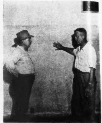
LLOYD H. YEAGER, general manager of the Gypsum Association (right) examines plastered wall in the Jayhawk Junior motel with Harry Lose, hotel official. Flood water level is apparent above the heads of Lose and Yeager. While water and mud stained the plaster, it failed to damage the wall otherwise.
