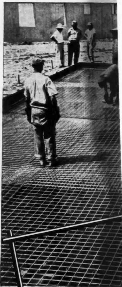
This picture shows American Welded Wire Fabric adding the high tensile strength of steel wires to a concrete ground slab. This type of construction protects the home against excessive settling and cracking, and insures the value of the buyer's investment.
