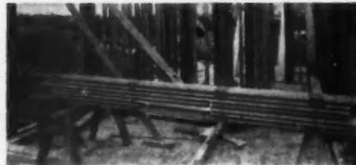
Frame delivered to the job pre-cut and fitted (above). A carpenter can nail together a 9-light window wall in 20 minutes (below).
