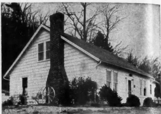
"CONCRETE CLAPBOARD" home of Victor Burkard, Barton, N.Y., whose blocks have 1/2-inch bevel on front to give clapboard effect
