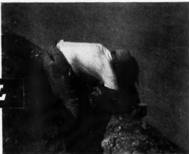
Al Loreti applies 2 coats of Thoroseal to concrete block foundation, as sure protection against rain and dampness.
