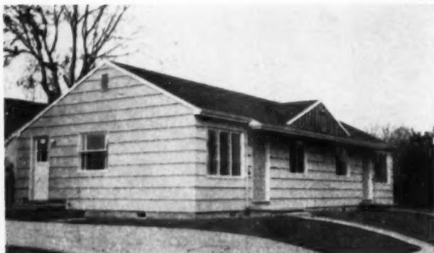
1,200 square feet of space, counting both units. Siding is cedar shakes. Hardwood floors and dry wall construction inside. The building is placed on a lot 50x100 feet
