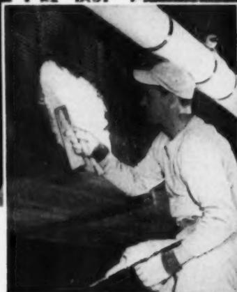
54,000 sq. ft. of plaster with Permalite were used to fireproof steel not only in General Assembly Building but also in two meeting halls. Plaster was applied 1" thick on expanded metal lath over steel beams, girders, trusses.
