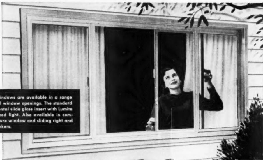
Rusco Horizontal Slide Windows are available in a range of sizes to fit conventional window openings. The standard unit consists of one horizontal slide glass insert with Lumite screen panel and one fixed light. Also available in composite unit with fixed picture window and sliding right and left hand ventilating flankers.
