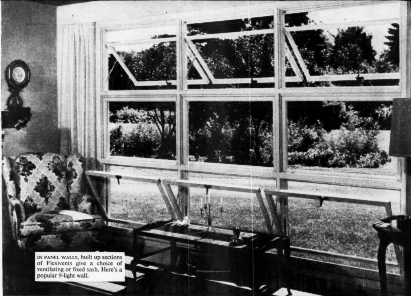
IN PANEL WALLS, built up sections of Flexivents give a choice of ventilating or fixed sash. Here's a popular 9-light wall.
