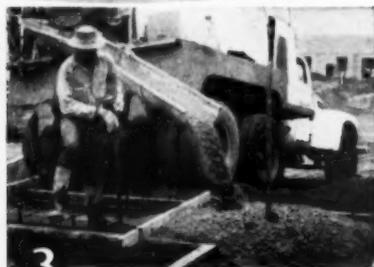
**3** Place concrete, using quality mix yielding durable walls. Use care to prevent honeycombing, especially along bottom edge.
