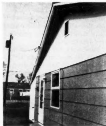
Closeup photo of rake shows construction. Ridge is extended two feet. Rake styling was copied from Al La Pierre in Seattle
