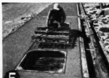
**5** Incorporate decorative designs before the concrete hardens. The illustration above shows workman adding a low-relief design.
