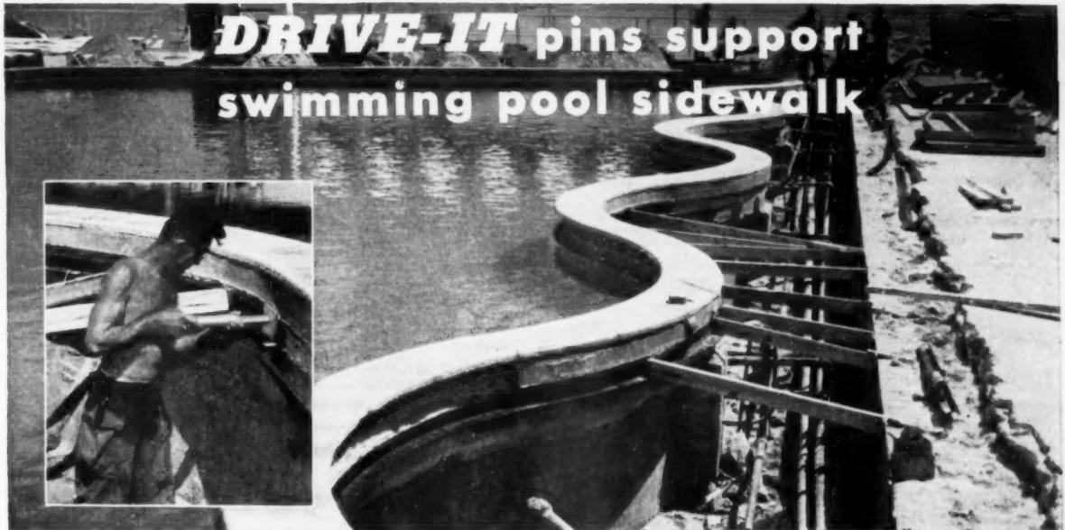
DRIVE-IT was used to help build a tunnel alongside the swimming pool at the Sans Souci Hotel, Miami Beach, Florida. The tunnel was needed to give workmen access to repair leaking pipes without the need of tearing up the sidewalk each time. The curved 1/4" angle iron was anchored to the concrete wall with DRIVE-IT. Cross (1/4" "I")
