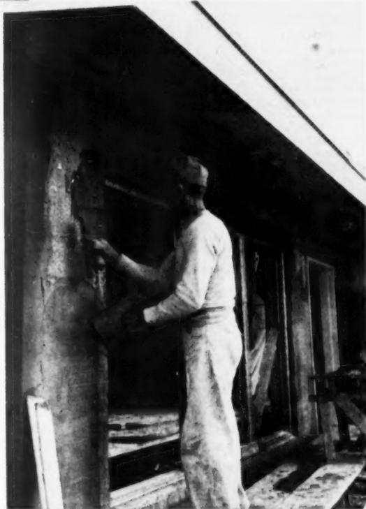
Workman is applying brown coat of stucco to block. A second coat followed by two coats of paint finish the exterior
