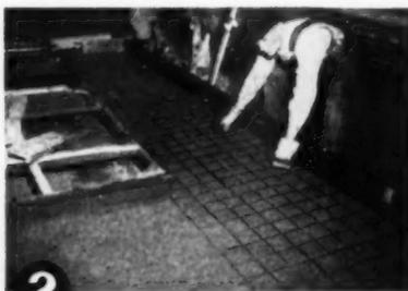
**2** Place the required amount of reinforcing in the panel and be sure to provide suitable means to hold it in the proper position.
