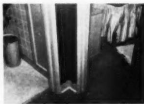
◀ Metal casing and Miami baseboard act as plaster grounds. Miami base is 16g material shimmied out 1/8 inch. Groove keys plaster for stability
