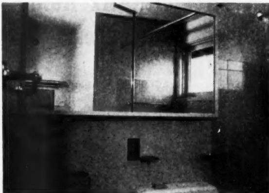
Large medicine cabinet has sliding mirror doors. Cabinet is shop built by builder. Mirrors are shipped ready for builders' installation
