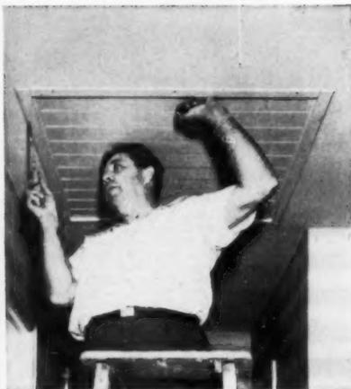
**Above:** Screw-fasten the automatic shutter to ceiling, with metal trim covering edges—no re-plastering.
