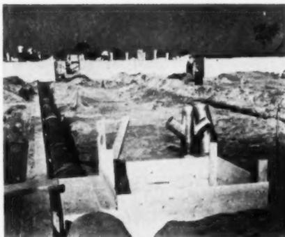
Layout of the heating system before the pouring of the slab shows the plenum form. As runs are unusually long, large diameter ducts are used. Reducing pipes as seen in the background serve branch lines from the plenum.
