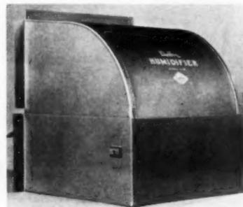
discharge of 3.9 pints of water per hour, a sufficient amount of moisture for the average installation. It circulates 85 cubic feet of air per minute. Powered by a fractional horsepower, moistureproof motor, the humidifier operates on 110 volt, 60 cycle, a.c. current. Daffin Manufacturing Co., Dept. AB, Lancaster, Pa.
