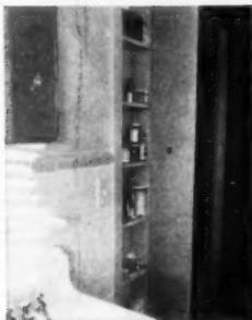
Between-the-stud medicine cabinet finds considerable storage use for many bath supplies. The unit fits between the studs, shelves are installed and a facing and door is applied
