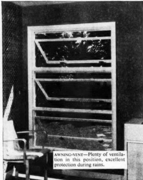
**AWNING-VENT**—Plenty of ventilation in this position, excellent protection during rains.
