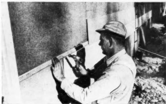
**3. Next, apply 1 1/4\" Shingle-Backer and asbestos-cement shingles.** System is self-aligning. No special nails or fasteners needed. Increases shingle exposure from customary 10 1/2\" to 11\" . . . gives 5% greater shingle coverage. Provides cushioned base to reduce impact breakage . . . reduces shingle waste as much as one-third. Increases insulation value of wall. Waterproofed throughout with asphalt.
