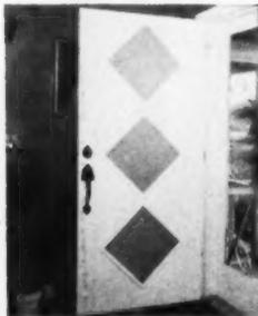
Diamond applique door is distinctive feature. Door is job built. Frame is 1x8's, interior face is 1/4-inch plywood, and exterior face is "V" groove cypress panel
