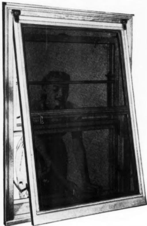
**EASY TO REMOVE.** The Andersen Storm-Screen hangs and opens like any standard screen or storm window.
