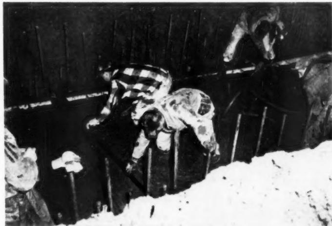
The concrete was screeded. Tarps were lowered and heat placed inside shelter during curing stage
