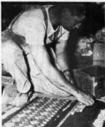
Making the ceramic tile facings for fireplace walls. (l. to r.) Each small tile is set by hand in small forms. Small sections are made into larger panels. Large panel is cemented to brick fireplace wall
