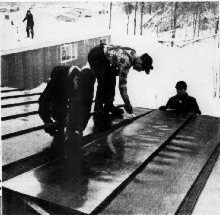
One roofer nailed flange to roof, another painted seam. Next panel was ready to position
