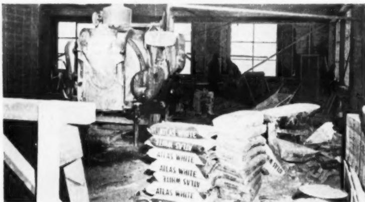
Mortar mixer was under cover in area warmed to 40 degrees to help batching
