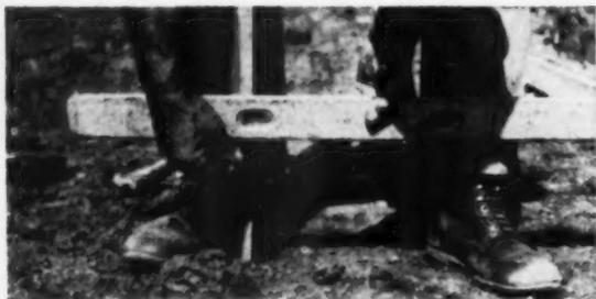
Setting stake for form in preparation for laying sidewalk. Grade of other form is established by means of a level
