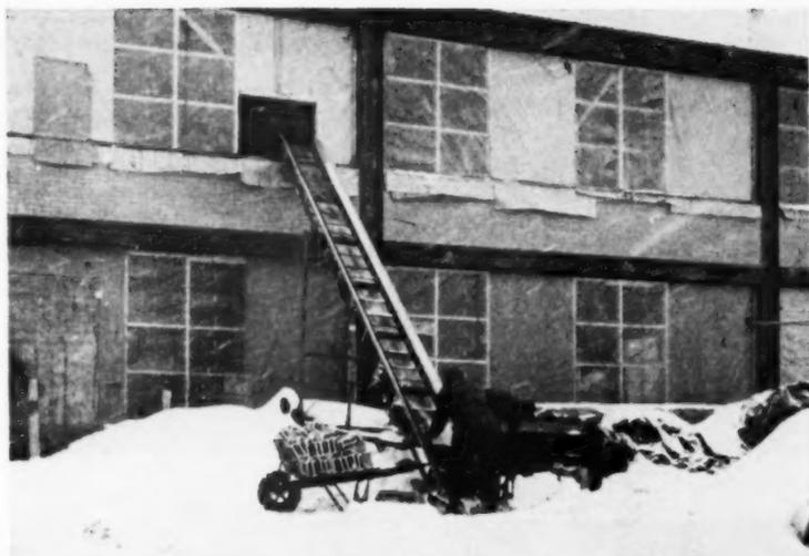
Portable conveyor carried hollow masonry units to second floor of office building. Note canvas cover for units stored in open
