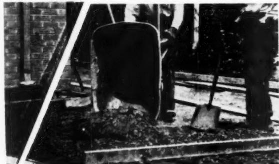
Concrete mix is poured and spaded against forms. Surface should be at least one inch above grade and pitched for drainage
