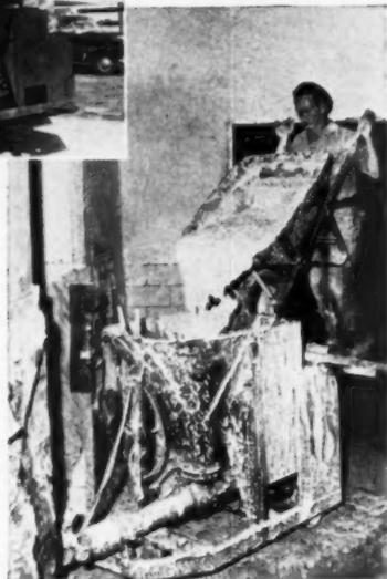
Truck-mounted or set up inside the building, the EZ-On machine pumps the wall material through a rubber hose from a hopper to a nozzle where compressed air creates a low-pressure spray
