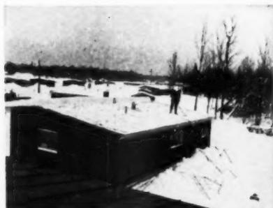
Roofer had to clean snow off roof before he could install standing seam terne plate. Extra man for snow removal, discarding of paper added to roofing cost
