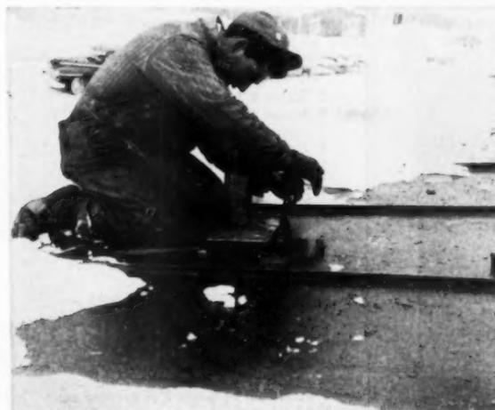
Lead vent flashing was prepared for soldering to terne metal
