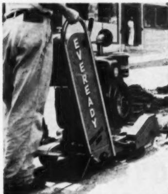
The saw is designed with a hydraulic control for lowering the blade at a controlled rate of speed as a means of providing longer blade life. There is no danger of bouncing the blade against the material.
