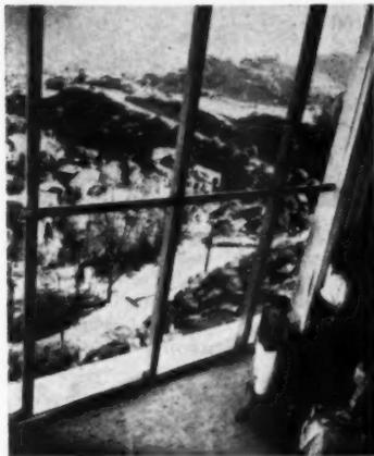
View through windows 18 feet high. Glass sections are 5x8 feet. One opens on ledge for window cleaning
