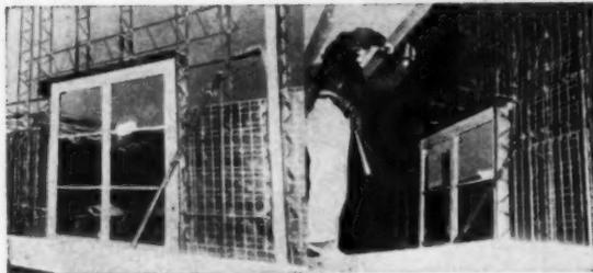
First a light steel frame of vertical wire trusses is erected. Paper-backed lath is wired on the outside of this frame. The procedure can be varied if conventional wood framing is used
