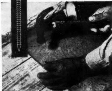
To make your linoleum underlays hold tightly and lie flat permanently, secure them with Hassall annular-threaded linoleum underlay drive screws. They are cement-coated for maximum gripping power. Heads are flat countersunk type. Size: 1/4" x #3 gauge. State quantity when writing for prices to:
