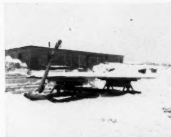
This bob-sled with tractor hitch was used to deliver lumber materials when roads were impassable to wheel machines
