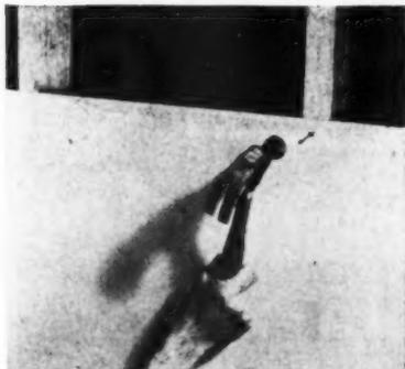
**Better nailability.** Fiberglas-reinforced gypsum board is less brittle, doesn't flake as readily during nailing. Nails hold better, too; reduces likelihood of unsightly pop-ups by nailheads. Installations look better . . . longer.
