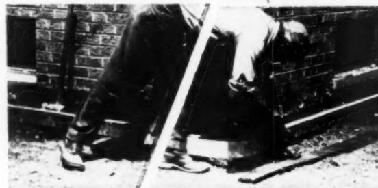
Tamping subgrade and constructing forms enough to hold concrete in place are preliminary steps in laying a driveway
