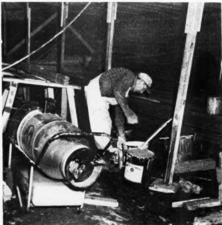
Silent Glow oil burner provided temporary heat in painting shed
