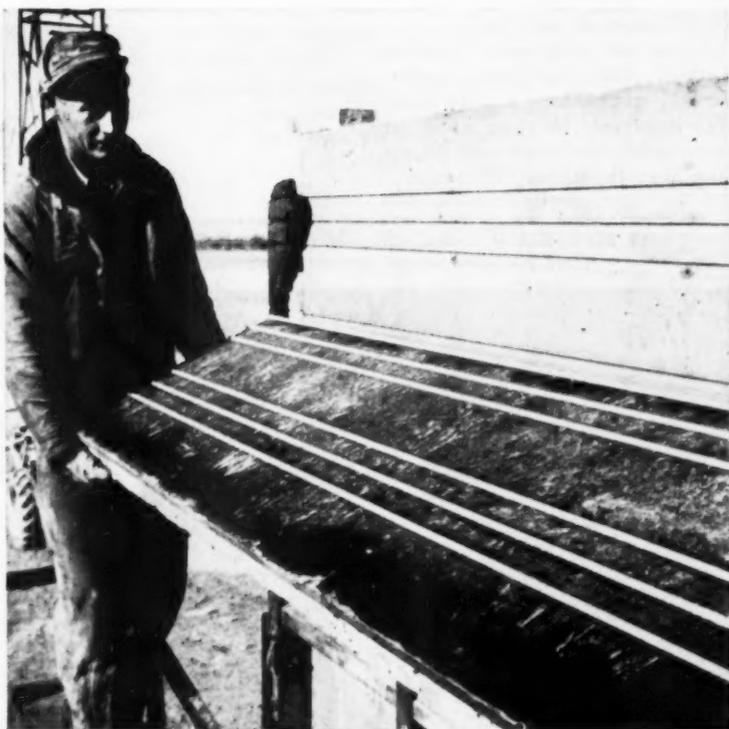
Scoring in the face of the exterior wall is made by aluminum half rods attached to the face of the form
