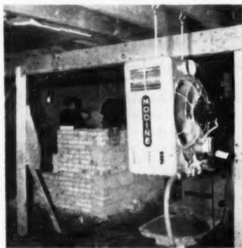
fired unit is light enough to be transported in the trunk of an automobile and can be installed without difficulty. It can be hooked up with temporary electrical wiring and a few feet of rubber hose to supply gas to the unit. Suspended from hooks screwed into a floor joist, it can be moved to other locations being worked on wherever heat is required. Modine Manufacturing Co., Dept. AB, Racine, Wis.
