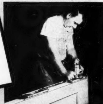
Router base and motor used with templet for cutting mortises. Provides perfect fit for round or square corner hinges. Accurate, micrometer depth adjustment.
