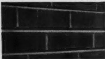
**True, tight joints** — Experience proves that masonry units are strongly bonded with Atlas Mortar; satisfactory hardening and tight joints are obtained.
