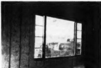
Rigid Styrofoam insulation is mortared to interior wall. Plastering is done over the Styrofoam
