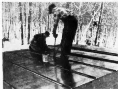
Standing seam was crimped to make it watertight and to hold it in position. Material had a base coat of paint
