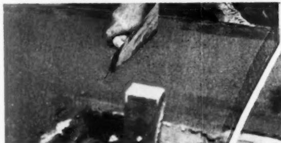
Trowel cut, about one third the depth of slab, is made at five-foot intervals. Cut is then edged with a grooving tool
