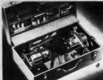
Stanley Builders Kit includes: 3/4 h.p. motor, straight and circular gauge, router base, plane attachment, arbor, plane cutter, mortising bits, templet guide, door and jamb buff templet, carrying case.
