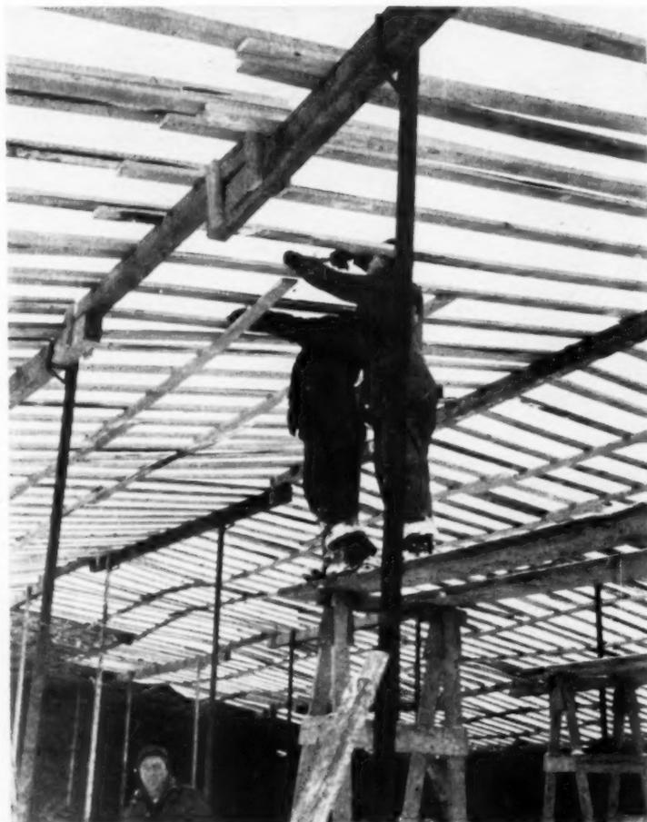
Shelters were built to protect concrete work. Tarps covered frame
