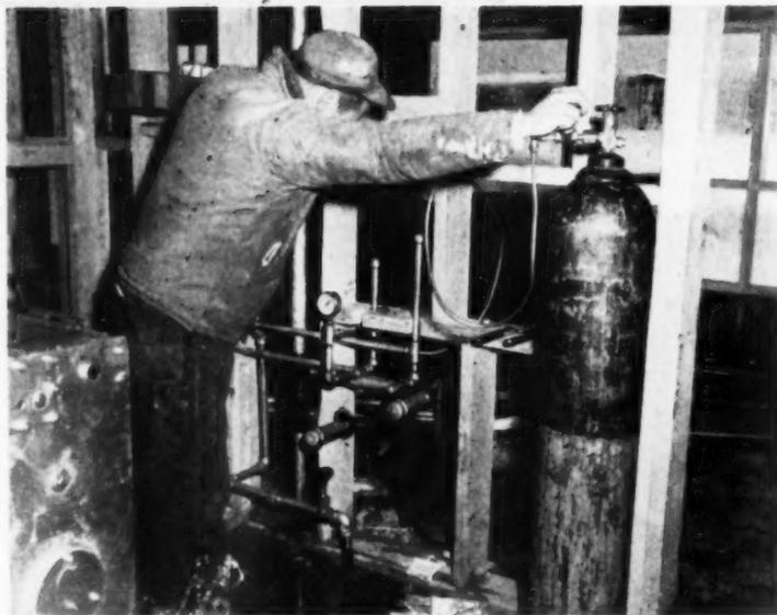
Nitrogen used to test service lines in place of water during winter. Tank had enough gas for four or five houses
