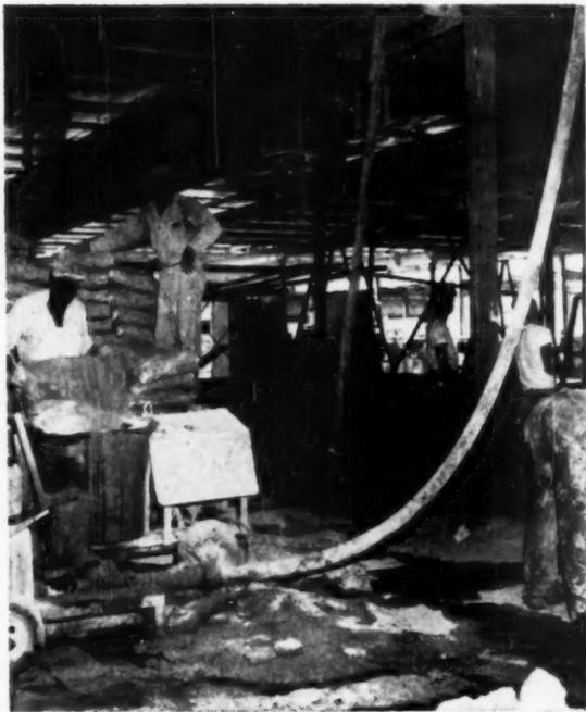
Pyrofill gypsum concrete is mechanically mixed and pumped from the ground level through a hose to the deck level
