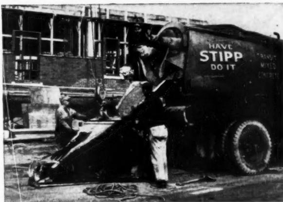
**POURING TRANSIT-MIXED DURAPLASTIC** concrete for Bell Telephone Dial Exchange in Olyphant, Pa. General Contractor: R. D. Richardson Constr. Co.; Ready-Mixed Concrete: Ezra Stipp Constr. Co., Scranton, Pa.
