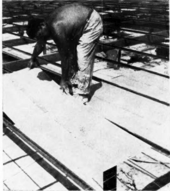
Gypsum formboard, 1/2-inch thick and 32 inches wide, is placed so that the end joints fall directly over the purlins
