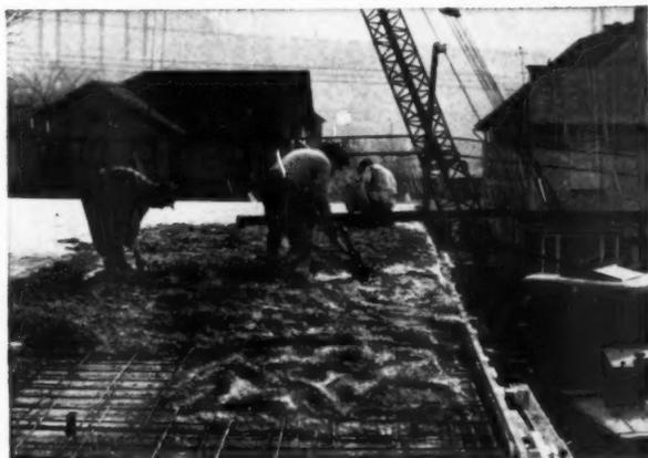
**WORKABLE CONCRETE** made with Duraplastic facilitates placement work in construction of this type. Workmen find it easy to place Duraplastic concrete properly around steel reinforcing.
