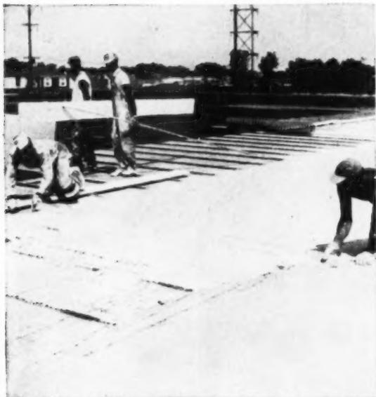
The gypsum slab is screeded immediately after pouring to a smooth, even surface
