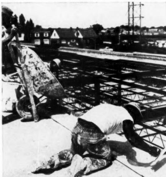
Finishing of edges is done by hand, and is an example of the clean character of the operation
