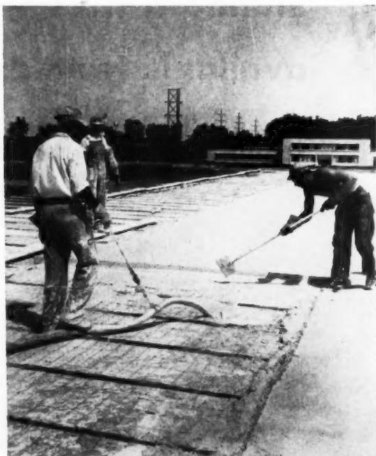
Caution is taken when pouring to make sure that the wire mesh is properly imbedded in the slab
