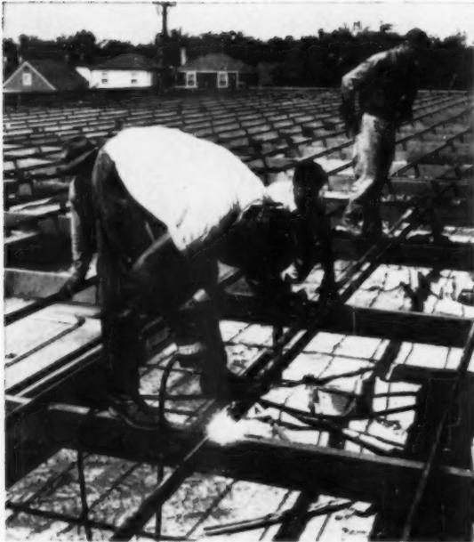
Sub-purlins are spaced accurately to hold the gypsum formboard. These are welded on alternate sides of each purlin crossing
