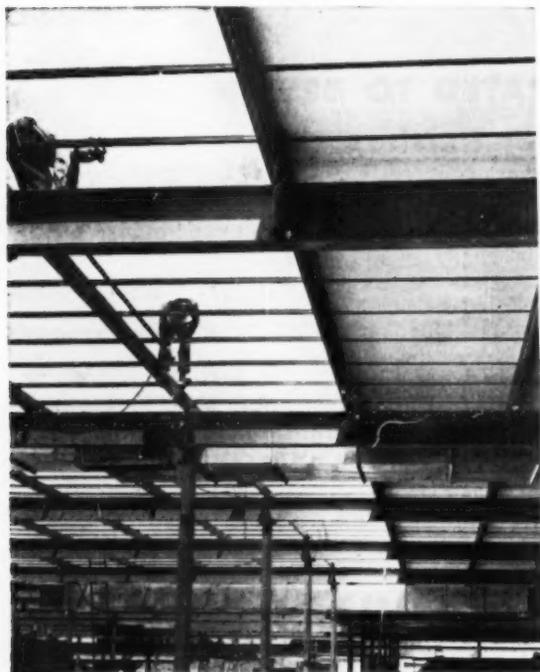
The interior of the job is kept clear of shoring. Erection is fast, and other trades are always free to proceed with their work
