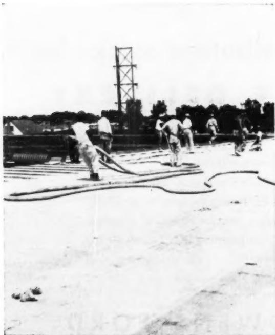
The pump and hose method assures quick pouring of the entire deck area. The slab can be walked on 15 minutes after pouring
