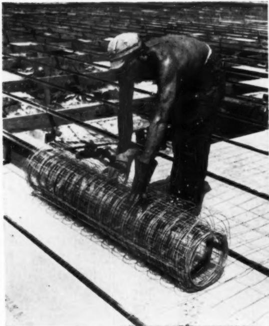
The welded wire reinforcing mesh is placed so that the rows of mesh touch, but do not lap at the edges
