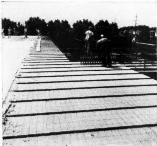
The formboard and the welded wire mesh are placed before pouring of the Pyrofill gypsum concrete
