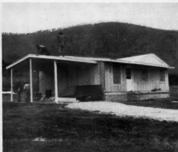
**4:30** Houses are erected and closed-in by seven-man crews in 8 hours, and are ready for interior finishing. Prime-coat painting of the exterior components safeguards them from inclement weather.
