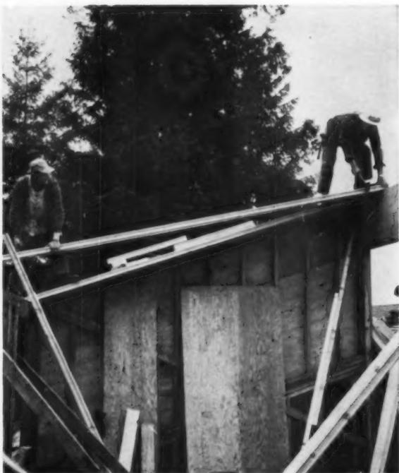
**Decking spans box beam and side walls**
