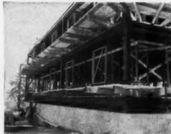
**STEEL-FRAMED** structure has 2-story-high wire studs, block foundation. Diamond lath goes inside. Mesh goes outside to hold stucco.
