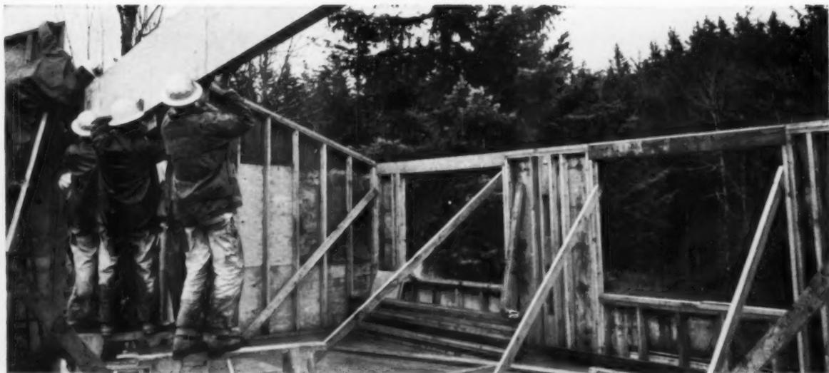
**Last phase: Lifting the lightweight box beam into place by hand takes only minutes.**
