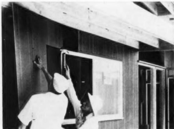
**Hardboard siding nailed right to studs**
