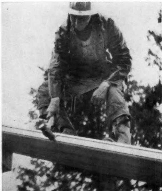
**Decking is pre-drilled for spiking**
