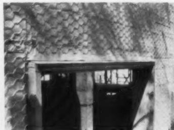
**CLOSE-UP** of Keymesh Lath that serves as base for 7/8" machine-applied marble-chip concrete. Wall is 3" of sprayed perlite concrete.
