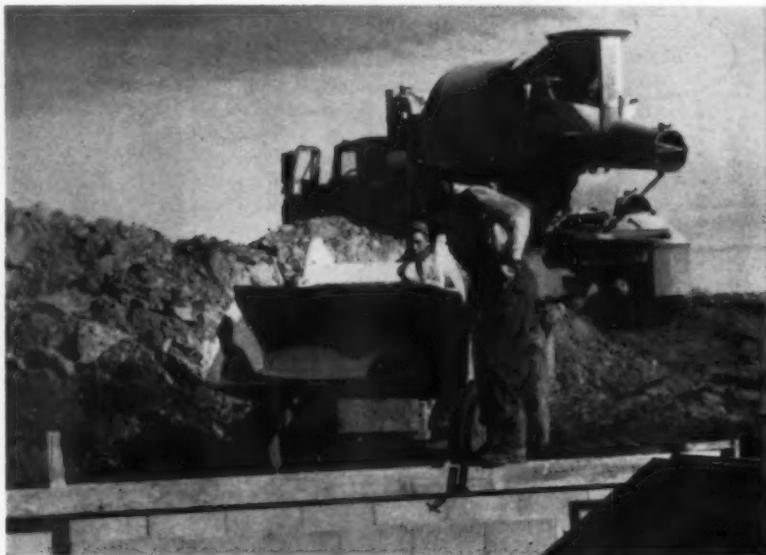
**Front-end loader takes concrete where mixer trucks can't go**
