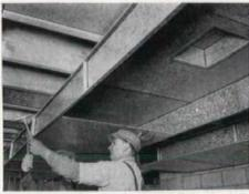
Even the trunks are standardized in the fully pre-fabricated Tempered-Aire duct system
