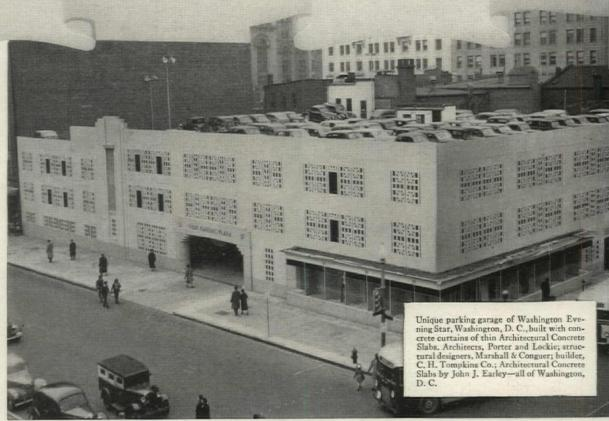
Architectural Concrete Slabs, hung from floors, provide decorative exterior walls with high structural strength, eliminate cost of fenestration and sprinkler system, save construction time, and allow adequate light and ventilation for a 3-story garage.
