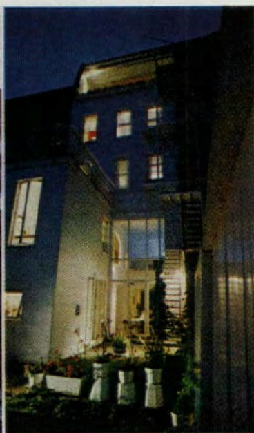
Front of classic old brownstone (far left) was left virtually as it was, but rear was drastically altered. Huge glass areas (near left) were installed in lower apartment and roof was cut back on top floor to create a terrace. Photos on these two pages show the lower apartment. Following two pages are of upper apartment.
