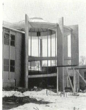
PRECAST CONCRETE FRAME
