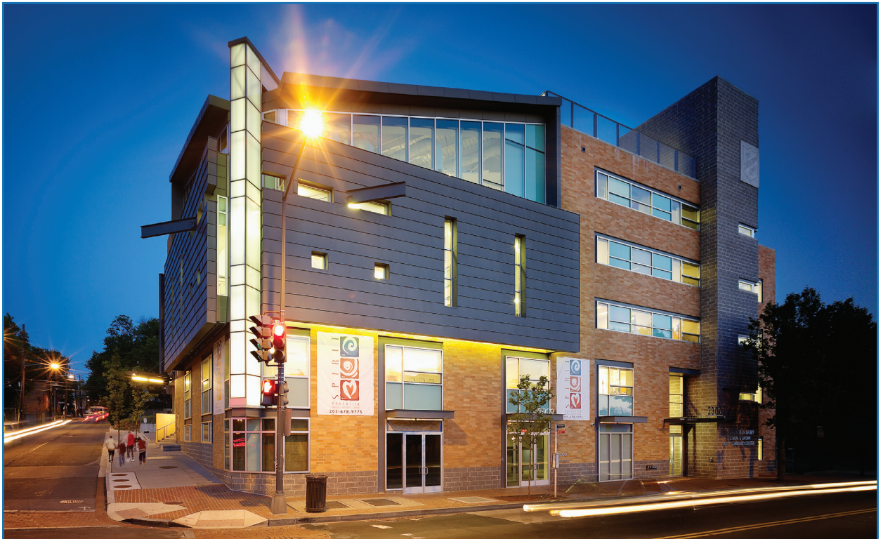
The Salvation Army center, with the cross on the corner rendered in back-lit glass and steel.
