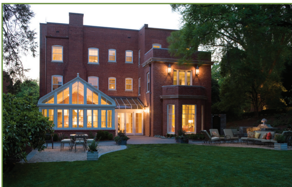
Rear façade of the house following renovation.
