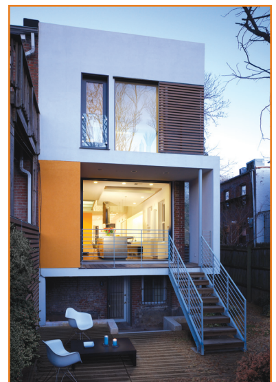
Rear façade following renovation.
