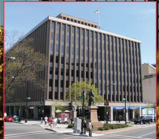
The building before renovation.
