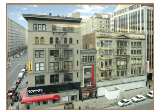
Photo by Shalom Baranes Associates Existing buildings before renovation.
