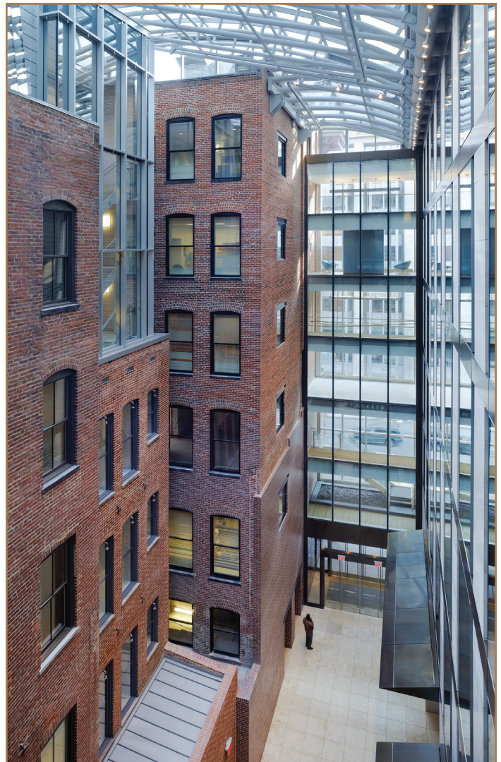
Atrium, with new office tower at right.
