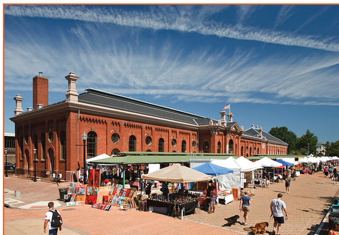
Eastern Market following the renovation.
