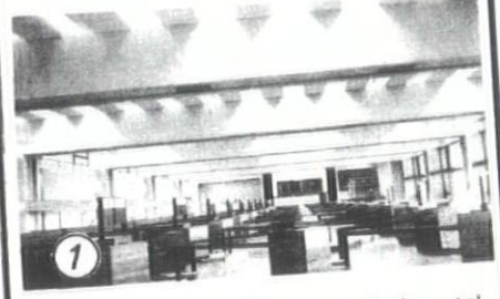
(1) Sprayed acoustic on vaulted metal lath shaped ceiling (New Departure Lobby-Upper Level)
