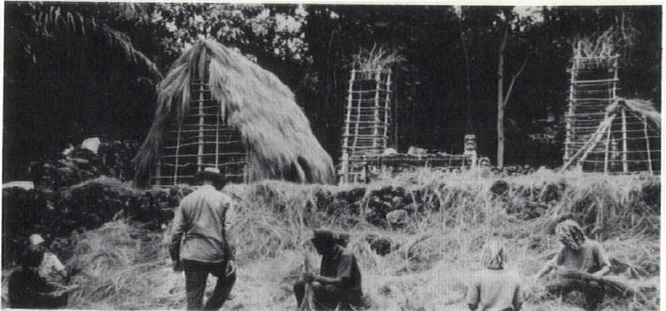
Partially completed pole-and-thatch structures on Kane'aki Heiau platform, during reconstruction in 1970.
