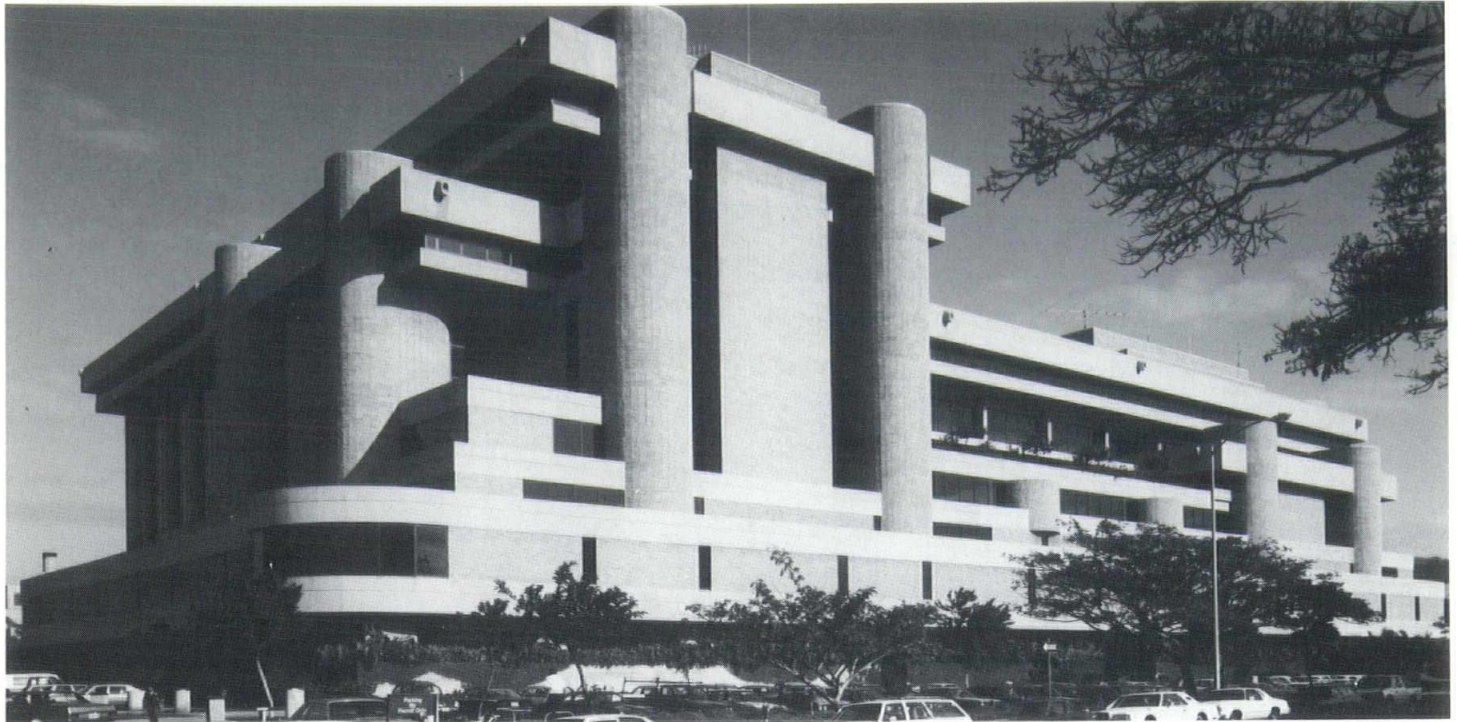
Completed in 1977, the Federal Building (photos on this page) has 629,000 net square feet of office space on nine floors, three courtrooms with judges chambers and other court related areas, and parking for 439 cars. Photos by David Franzen.
