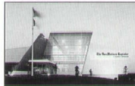
Des Moines Register Newspaper Production Facility
