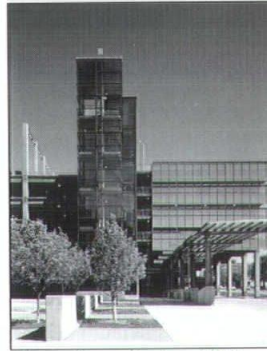
Center Street Park and Ride, Des Moines, Iowa
