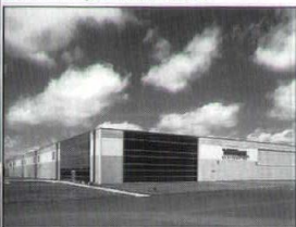
Visionaire Aircraft Assembly Facility, Ames, Iowa
