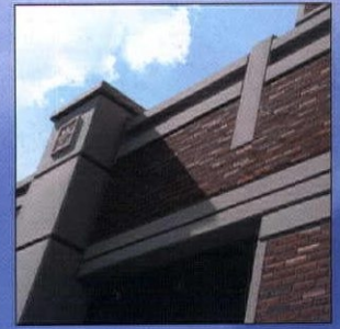
Zona Rosa parking deck Kansas City, MO
