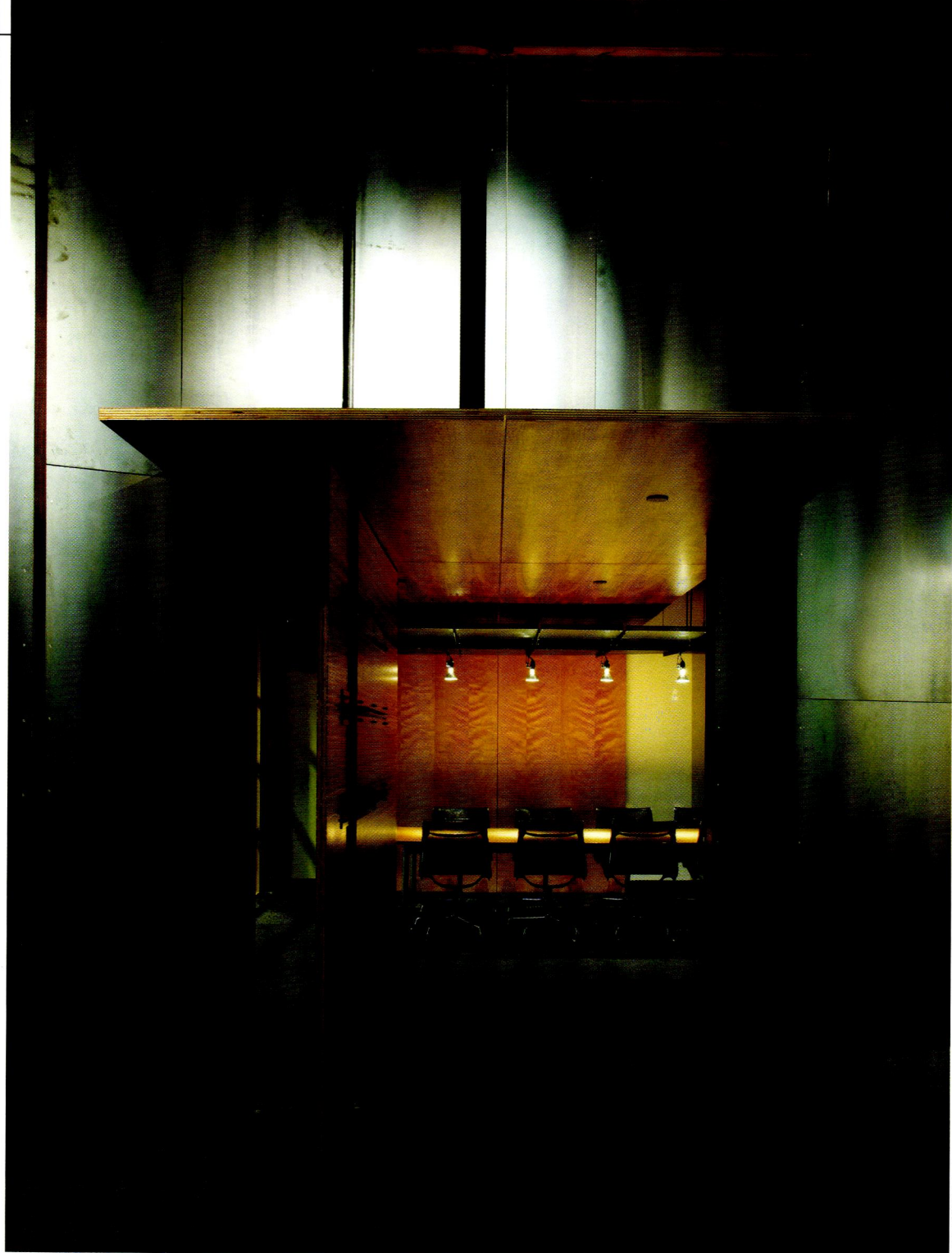
Left: The entry to the conference room is a large Plyboo door with a custom fabricated set of steel hinges. This is set into an angled steel wall that guides visitors from the lobby into the studio space.
