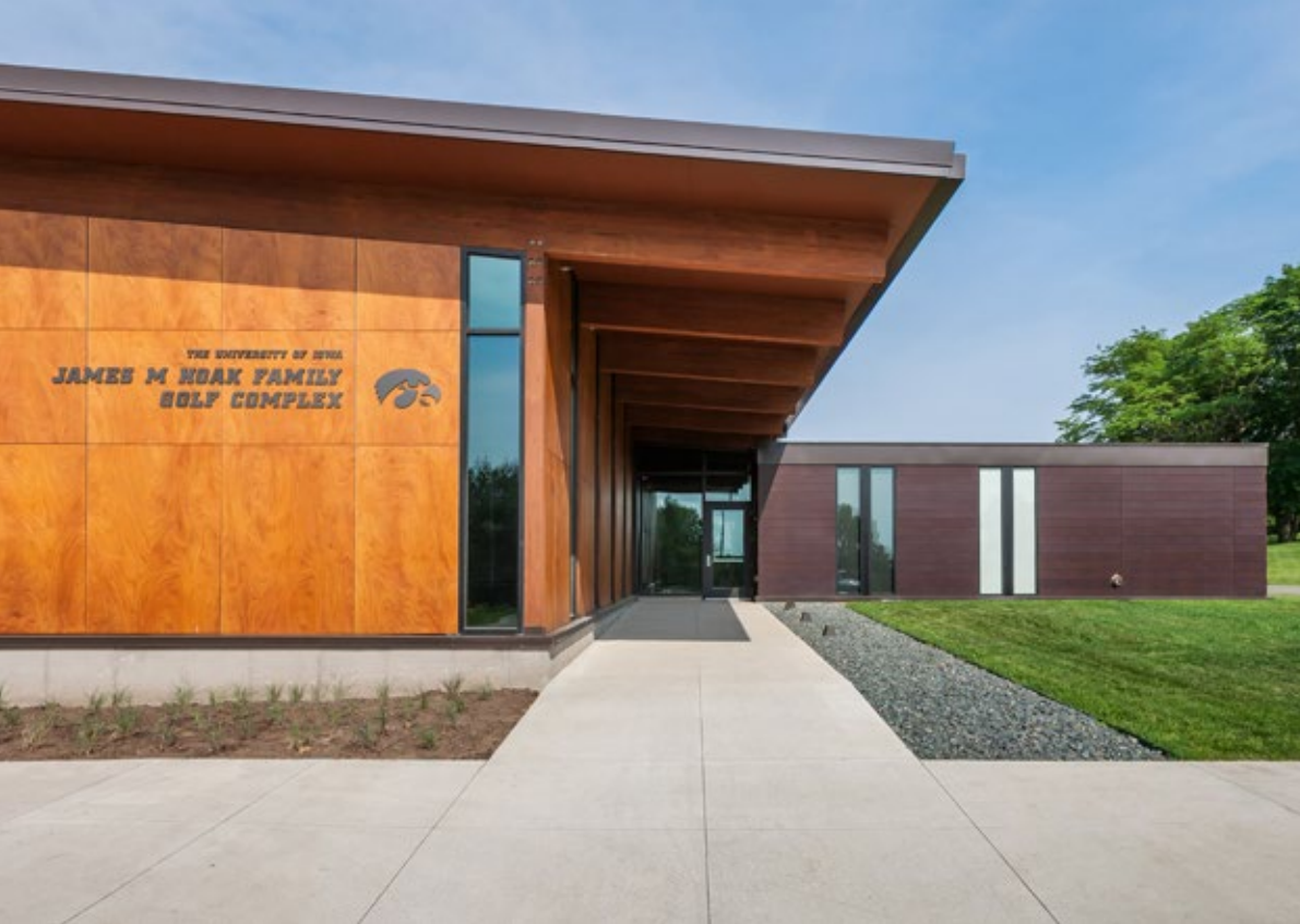
Left: Wide overhangs help to deflect the sun's intense rays; the building form to the right opens up onto the course.
