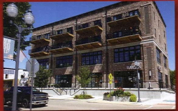
Newbo Station, Cedar Rapids Fusion Architects
