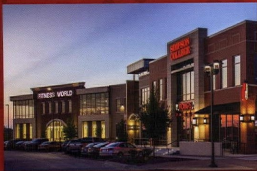
Vintage Main, Ankeny Imprint Architects Mason Contractor: Forrest & Associate
