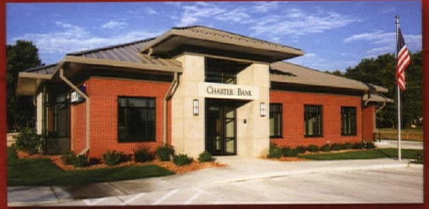
Charter Bank, Ankeny CMBA Architects Mason Contractor: Forrest & Associate
