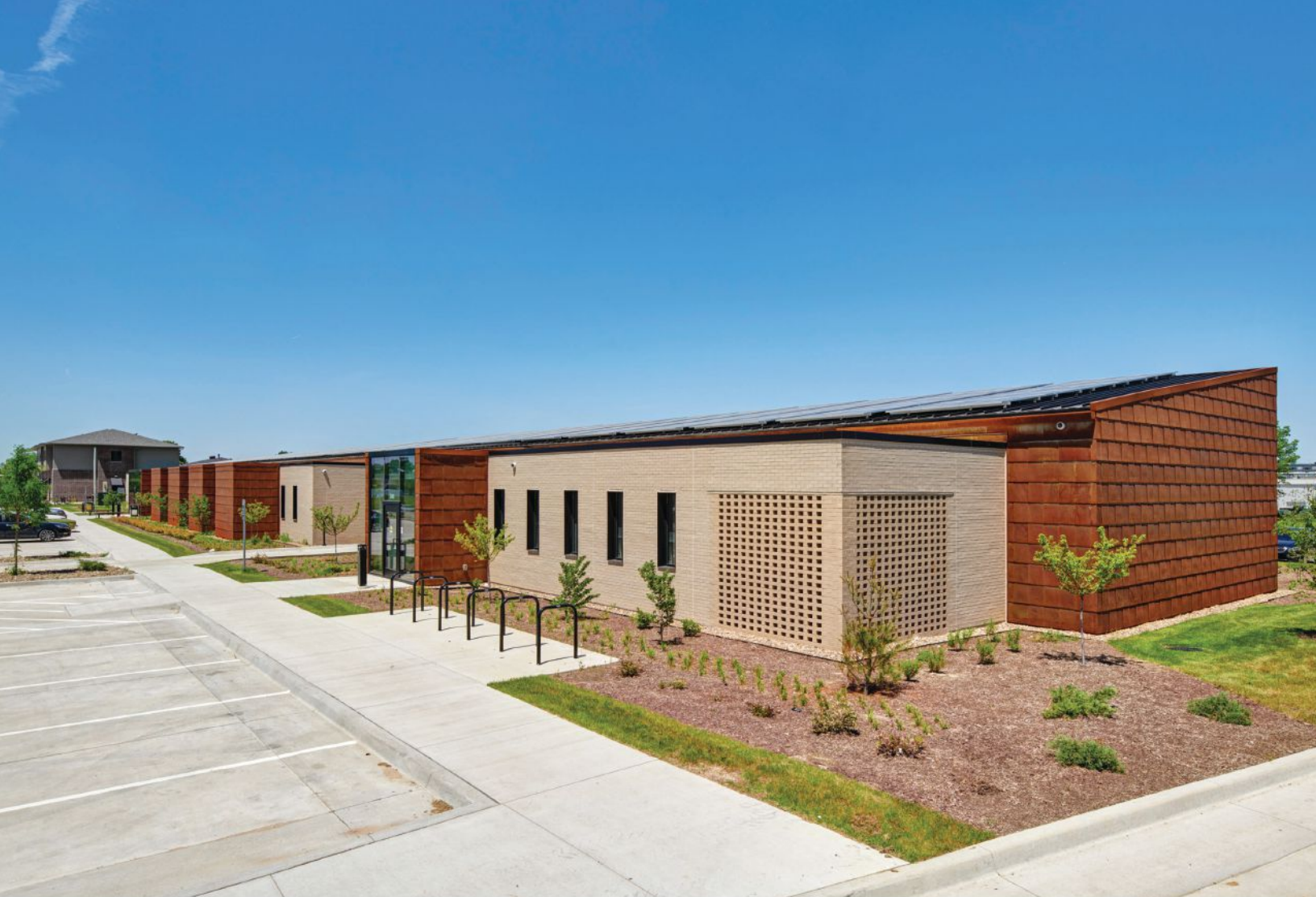
The building systems include a 390-panel solar array that is projected to offset over 50 percent of the building's total expected load.
