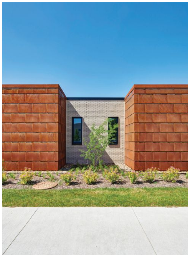
Windows are inset from the face of the building and granted additional privacy through landscaping.
