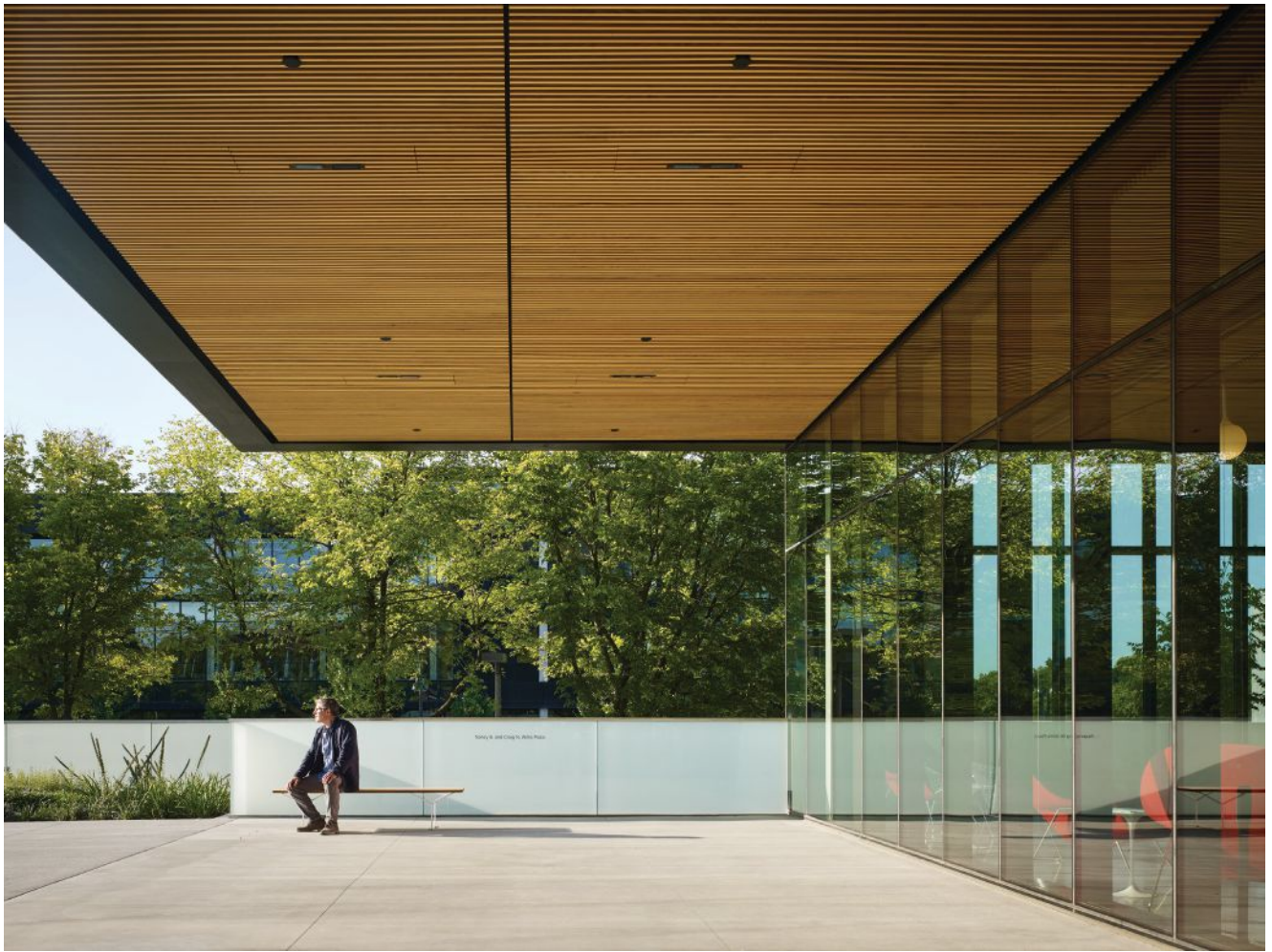
Above: Although the new building is also located near the river’s 500-year flood zone, its robust protection strategy will ensure that the museum’s contents stay safe and dry in another catastrophic event. Opposite: BNIM worked closely with the university during site selection to make sure the museum’s orientation, accessibility, and visibility would connect the campus and draw in visitors..
