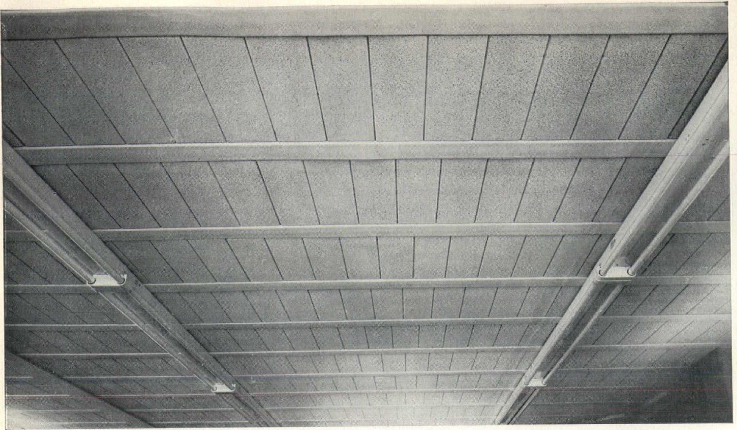
This acoustical ceiling-roof features the precast concrete TEE-BLOK JOIST System with attractive lightweight flush filler block.
