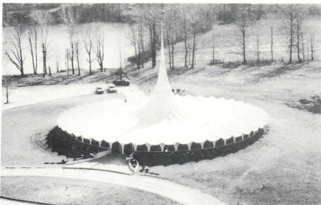
Region 6: First Christian Church, Brazil; Architects: Bozalis, Dickinson, Roloff, AIA, Oklahoma City; built in 1966.
