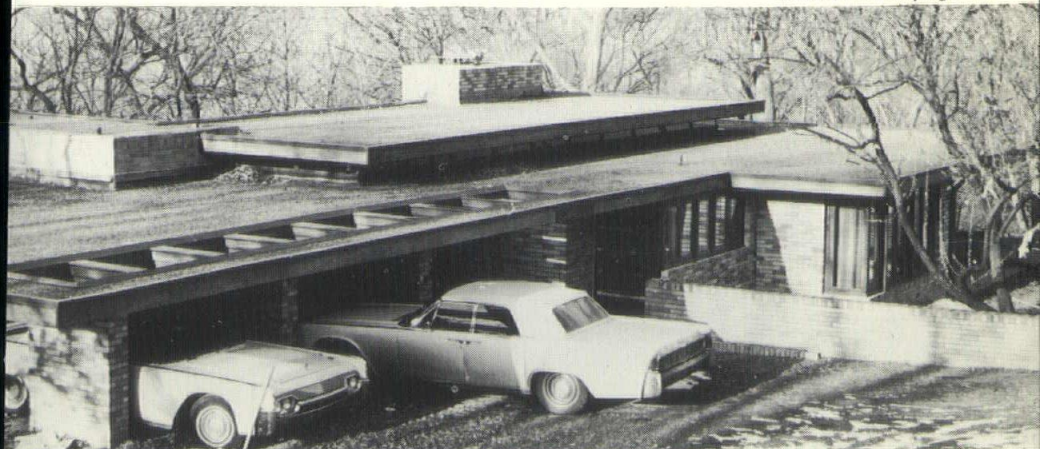
The entrance to the Sondern home at 3600 Belleview avenue, now owned by Richard Stern, is through the shadows of the port for three cars. In the center is the kitchen, and to the right the living and dining space.
