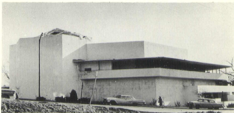
A lost opportunity, Wright's largest project here, the Community Christian church, stands bleakly in the winter sun. The structure was only about half completed according to the architect's plans, and later was defiled by additions. The loss is the city's, for in Wright's 89 years he designed only six or seven churches.
