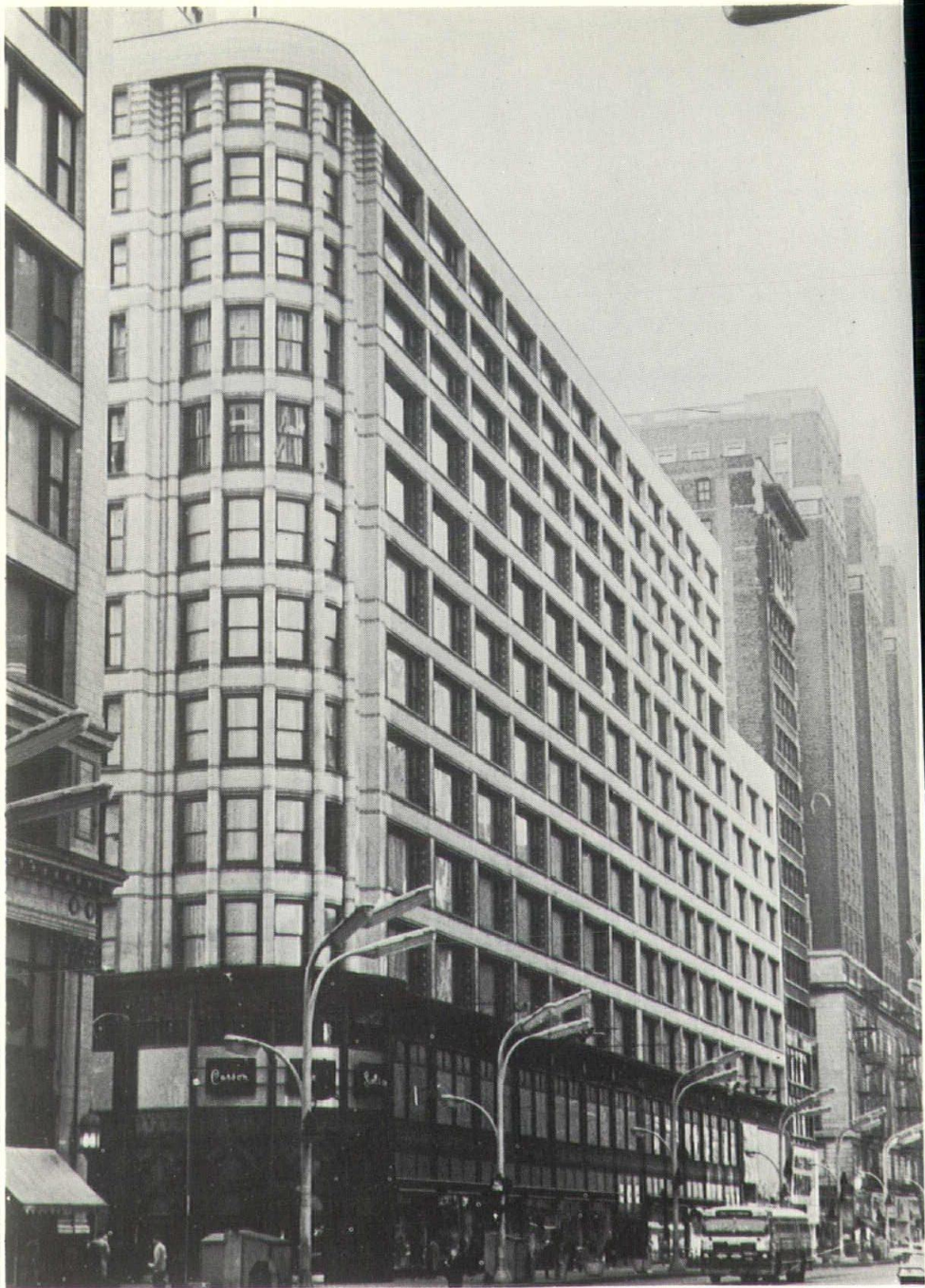
One of the great monuments of the Chicago School of steel-frame skyscraper construction is the Schlesinger & Mayer Department Store, now known as the Carson, Pirie, Scott Store. Here Louis Sullivan clearly expressed the framing on the upper floors and embellished the two-story base with cast iron ornament of almost incredible richness.
