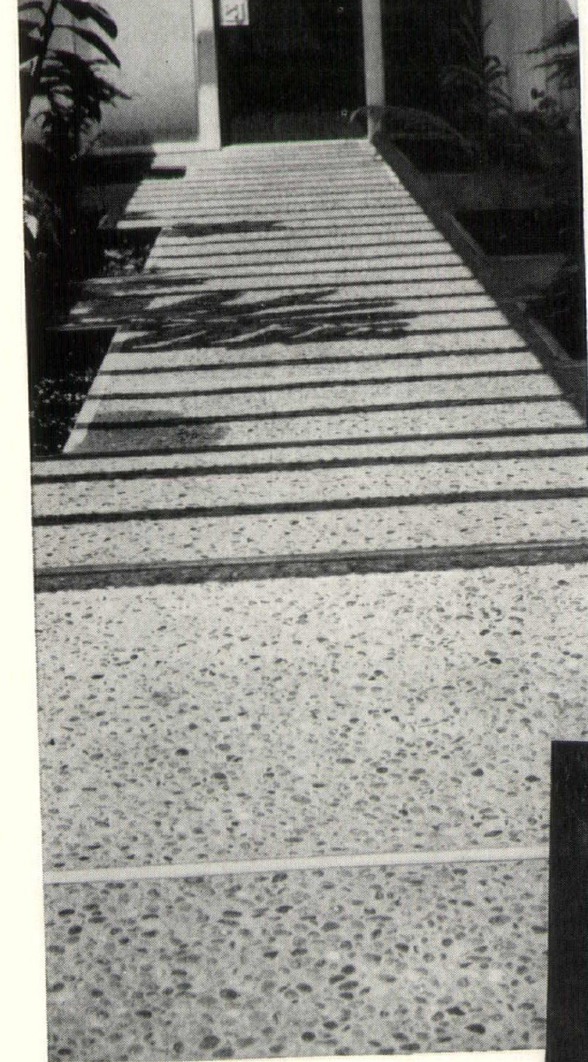
Pebbled concrete fits the modern approach. Landscape Architect: Richard Beeson.
