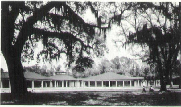
D. C. REEVES ELEMENTARY SCHOOL, Ponchatoula, La. DESMOND-MIREMONT-BURKS, Architects and Engineers ANDREW GASAWAY, Associate
