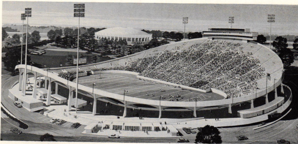
GENERAL CONTRACTORS FOR MEMPHIS' 50,000-SEAT STADIUM NOW UNDER CONSTRUCTION
