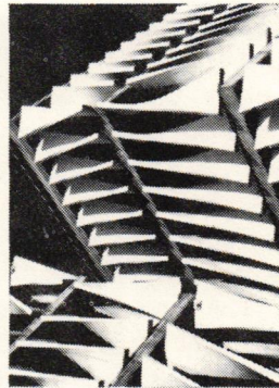
Movable forms were used for world's largest concrete dome. University of Illinois Assembly Hall. Architect: Harrison & Abramovitz. Structural Engineers: Ammann & Whitney, New York
