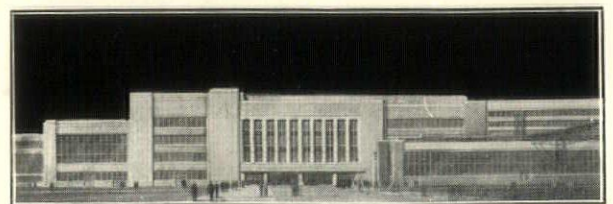
Press Shop, Ford Rouge Plant, East Elevation
